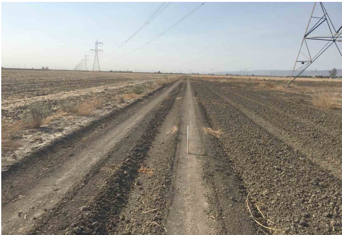
Photo No. 2 High Voltage Transmission Line Easement (between Phases 5 and 6)
