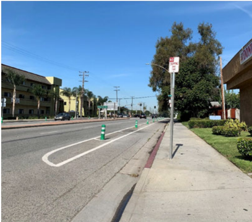
Protected (Class IV) bicycle lane on Wardlow Road, west of Pacific Place (westbound direction) (Photo Credit: Fehr & Peers, September 2020).
