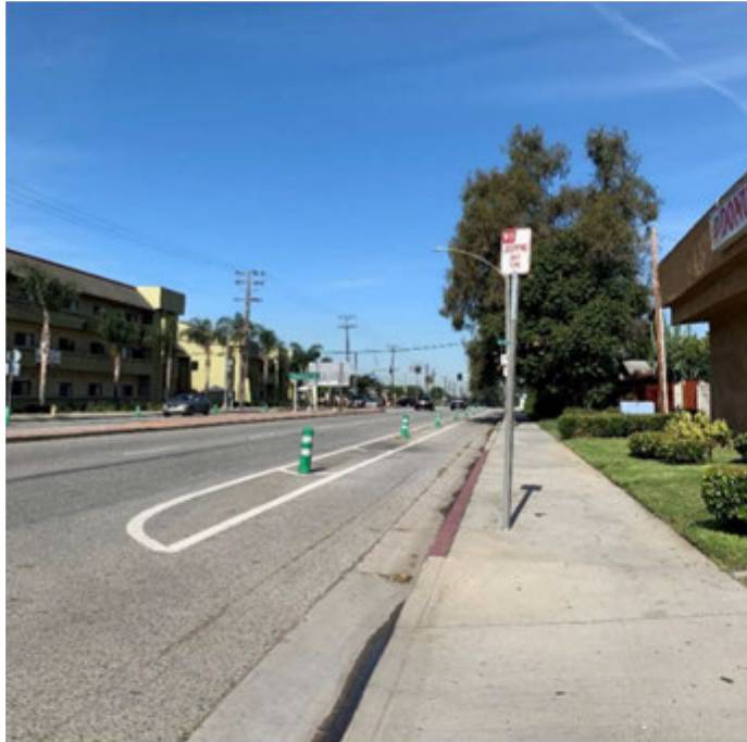
Protected (Class IV) bicycle lane on Wardlow Road, west of Pacific Place (westbound direction). (Photo Credit: Fehr & Peers, September 2020.)
