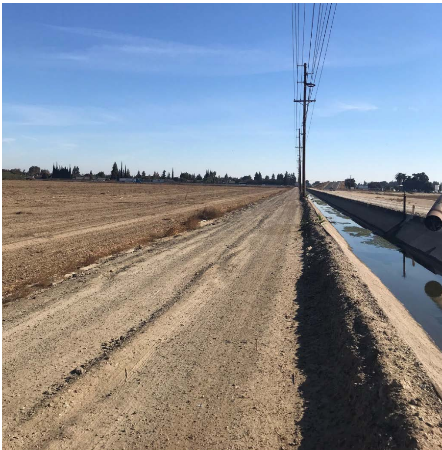
View east long TID canal and TID access road from Dianne Drive. Project parcel is on the left, outside of the TID right of way. November 10, 2020.
