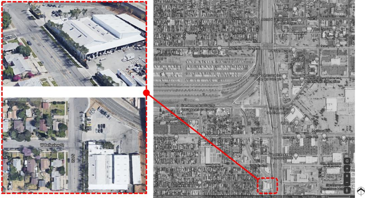
Figure 7 – Representative Pre-Engineered Steel Frame Building (Type #1)
