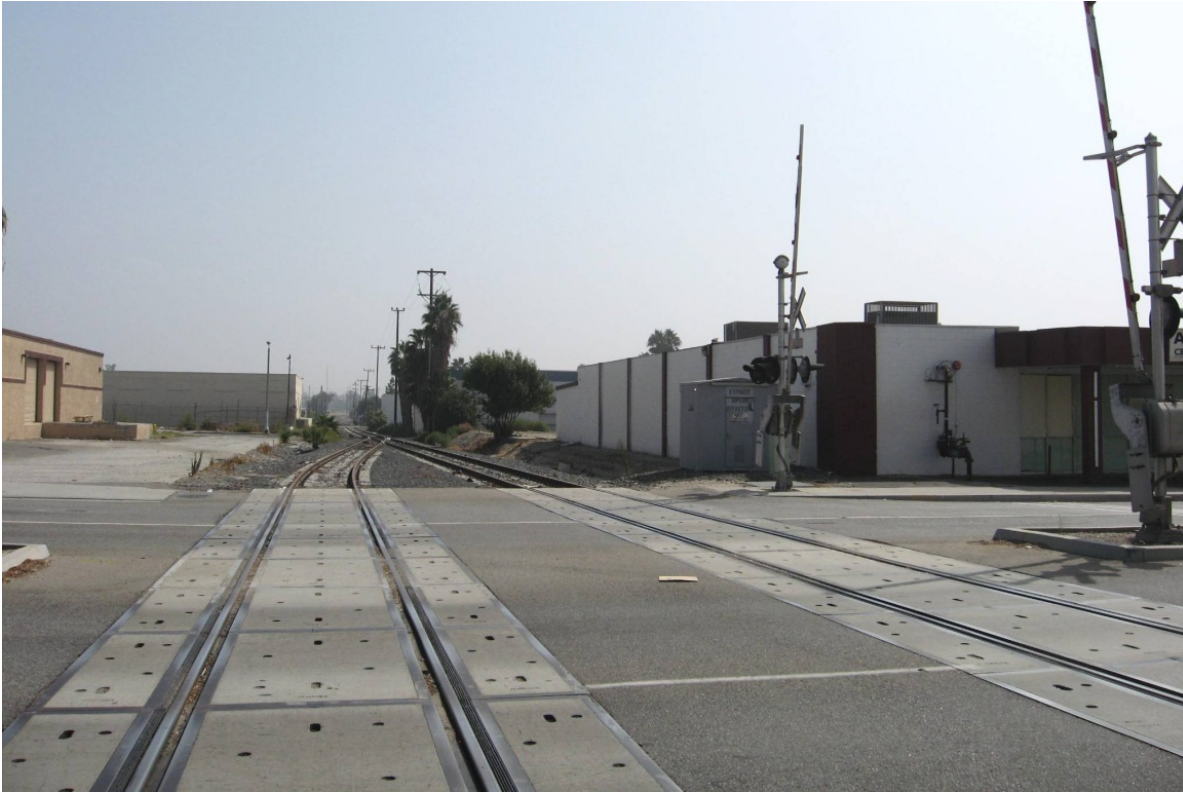
Figure 3.2-18 (VP K): Looking East, E Street at Railroad Crossing
