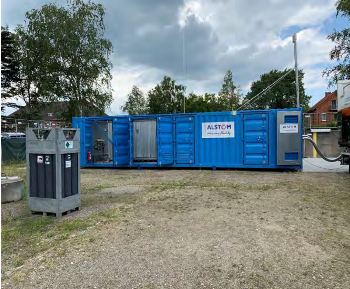
Figure 7. Liquid to Gas Conversion Container
