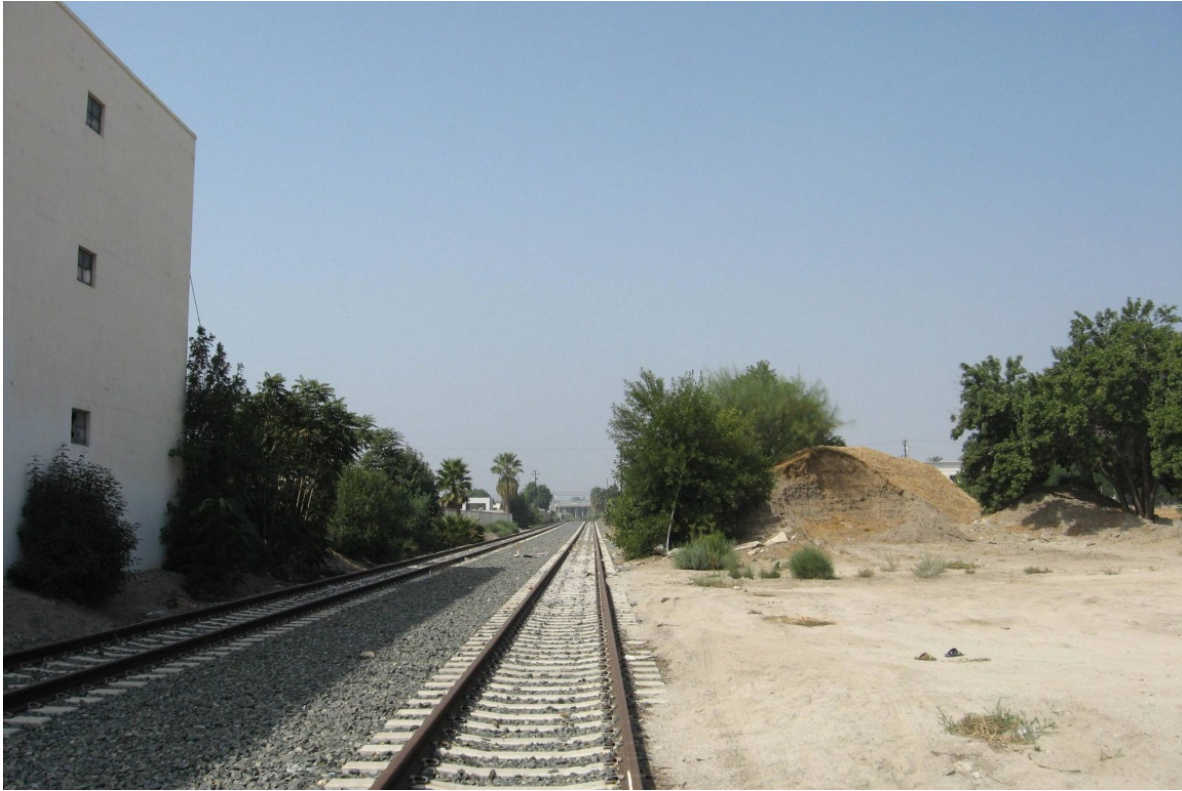
Figure 3.2-19 (VP L): Looking West along Railroad Right-of-Way at E Street at Bus Facility Site
