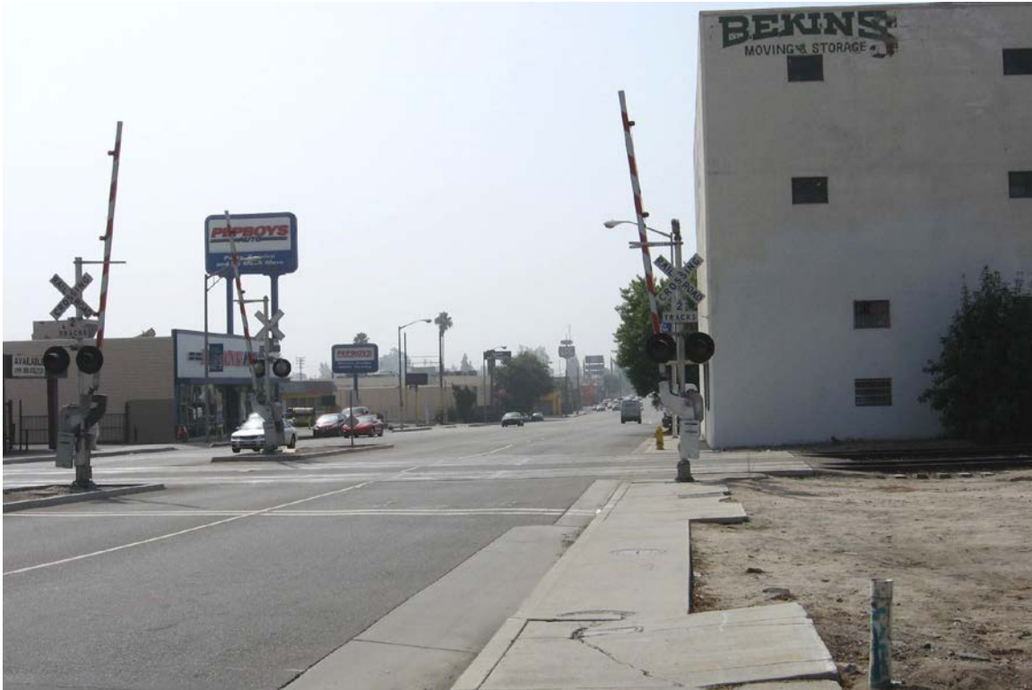
Figure 3.2-17 (KOP 5): Looking South, E Street at Railroad Crossing/Bekins Moving and Storage at Bus Facility Site
