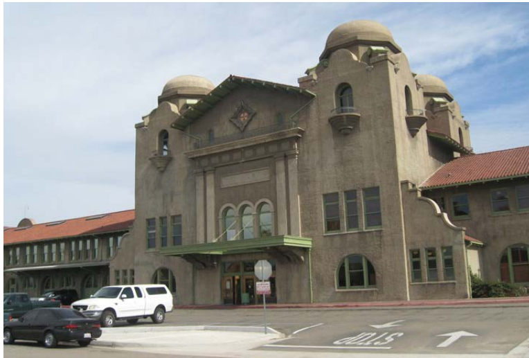
Photo 4.6-4. Front Façade of the Depot
