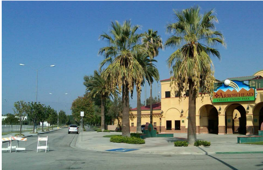
Photo 4.6-3. Closed Access to the Affected Area within the Project Study Area
