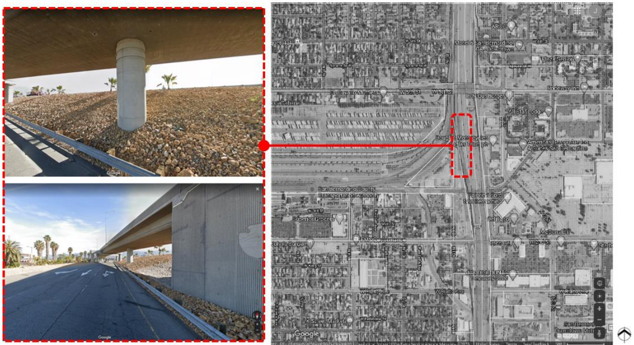
Figure 10 – Elevated Roadway Segment
