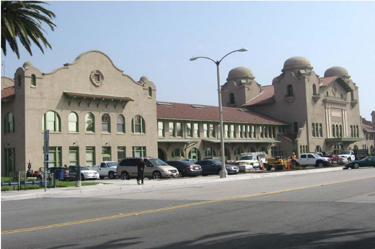
Figure 3.2-5 (KOP 2): Santa Fe Depot Building, along 3 rd Street Looking Northeast
