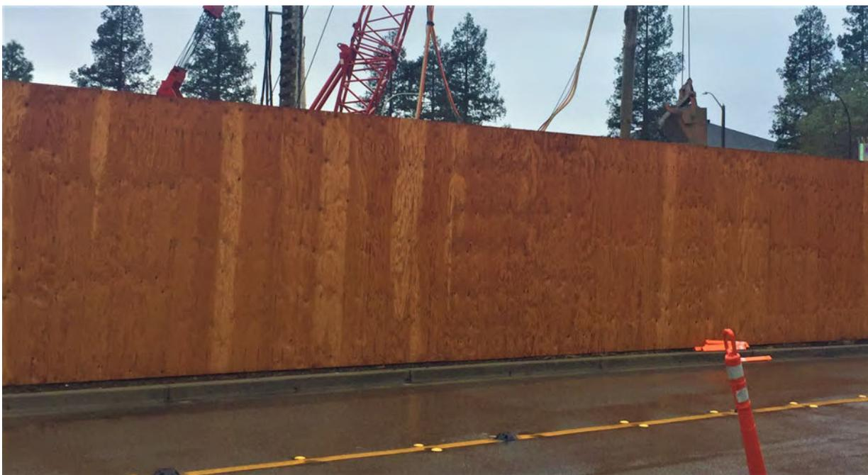
*Top: 10-foot-tall barrier consisting of double ¾" plywood affixed to 6 x 6 posts driven into the ground. Bottom: Solid exterior face of the same 10-foot-tall barrier. Image Source: MIG.*
