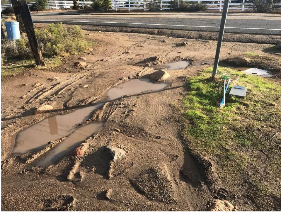
Photo 1. (12/7/18) View facing northeast of Basin AP-001. The basin is a series of ruts that was regularly disturbed by vehicle traffic. This photo was taken during the first sampling visit to the Alpine site.
