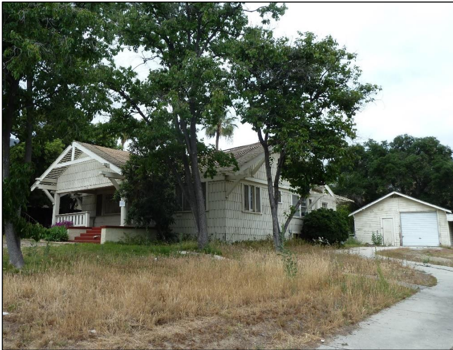
Photograph 1: West and south elevation of dwelling with detached garage, camera facing northeast. City of Glendale 2016.
