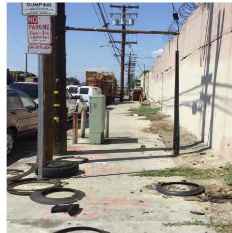
Industrial street with approx. 8 ft. sidewalk and utilities that conflict with clear walking path
