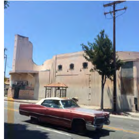
Gentry Theater | Source: A Paseo Through Time in Florence Firestone
