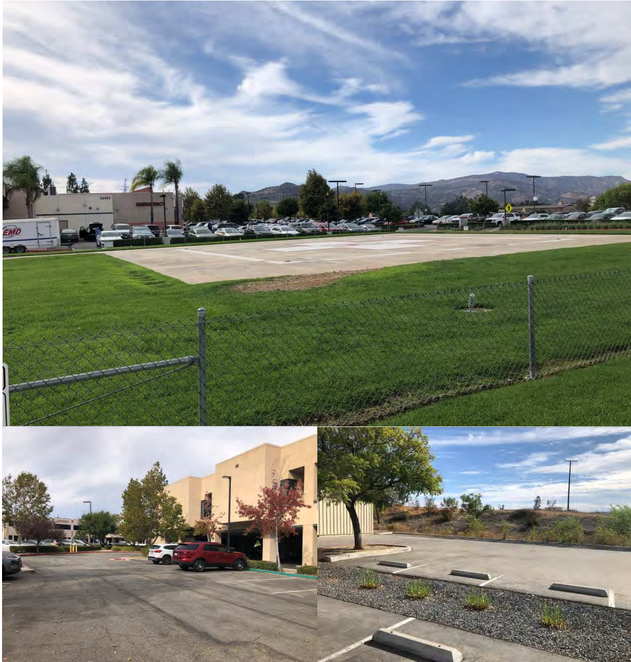
Figure 4. Overviews of the existing development at the Project site. Top: View facing southeast toward existing Building B-H, with the ground-level helipad visible in the foreground. Bottom left: View of the rear of existing Building I. Bottom right: View of the southern parking lot facing south towards I-15.
