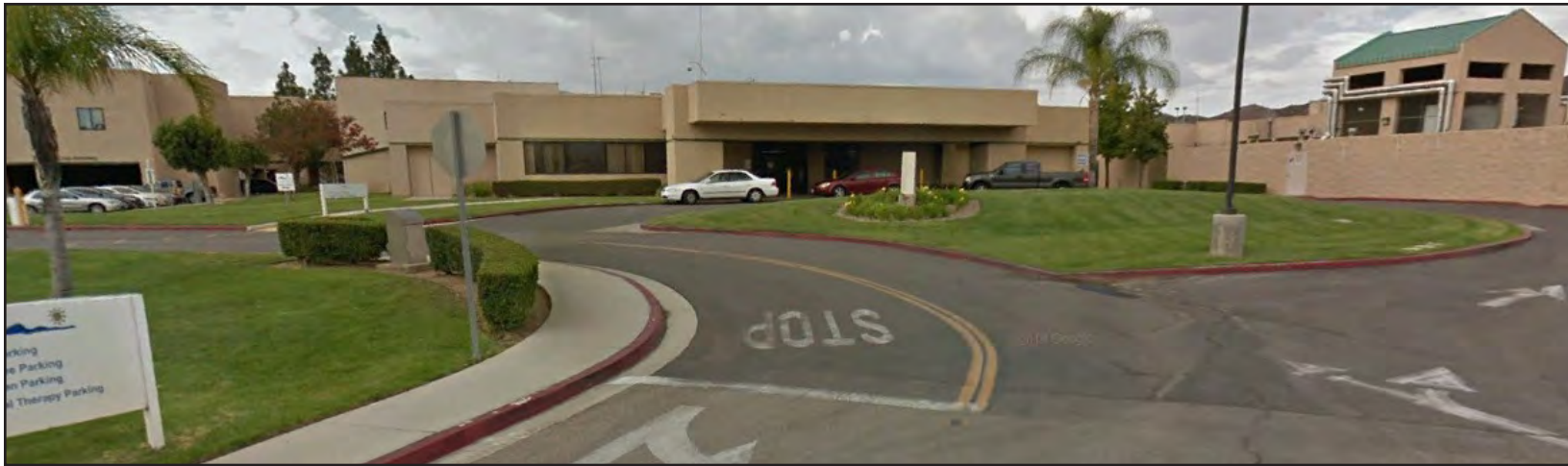
Photo 3. View from Parking Lot off of Prielipp Road.
