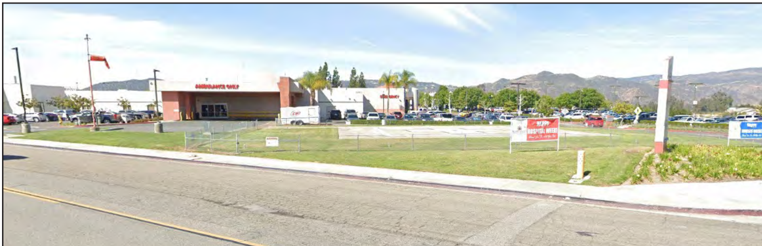
Photo 4. View of Existing Helipad from Inland Valley Drive.
