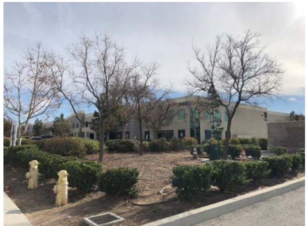
48. View of the adjacent multi-tenant buildings to the east-southeast.
