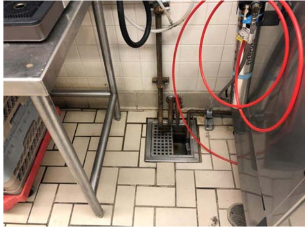
32. View of the kitchen floor drains.
