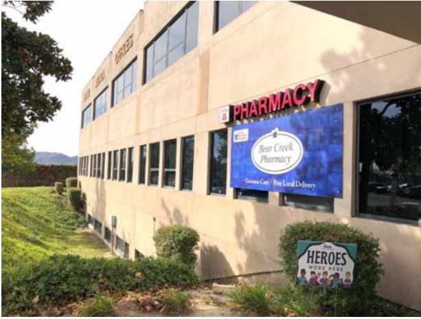
37. View of the three-story office building on the northwest portion of the site.
