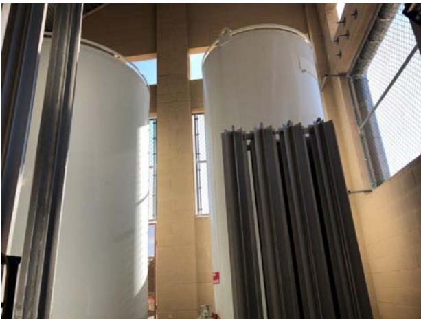
15. View of the liquid oxygen ASTs.
