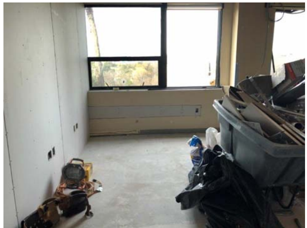
40. View of ongoing office tenant improvements.
