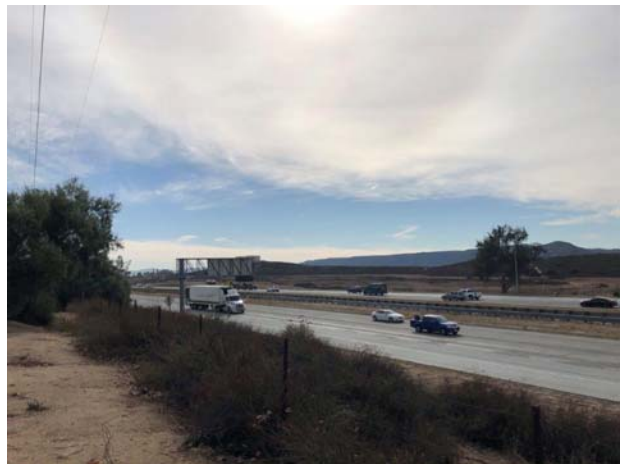
46. View of the freeway to the west.
