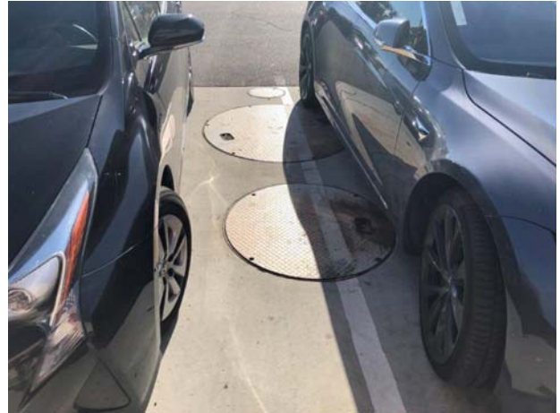
20. View of the decontamination UST.
