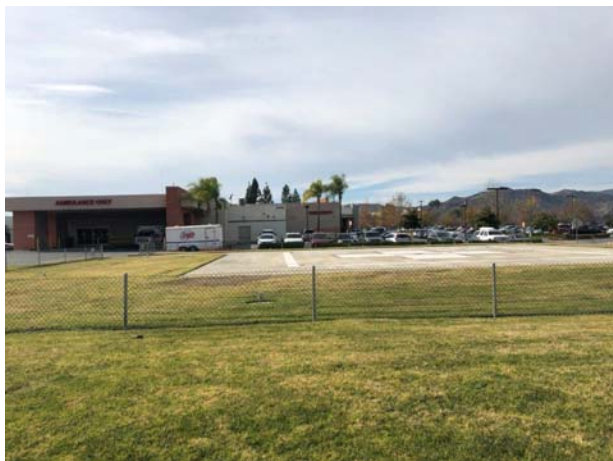
5. View of the helipad on the northeast portion of the site.
