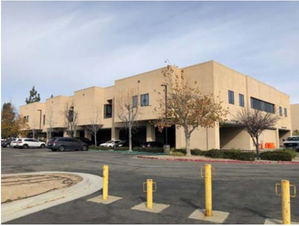
7. View of the subject property west wing, two-story building.
