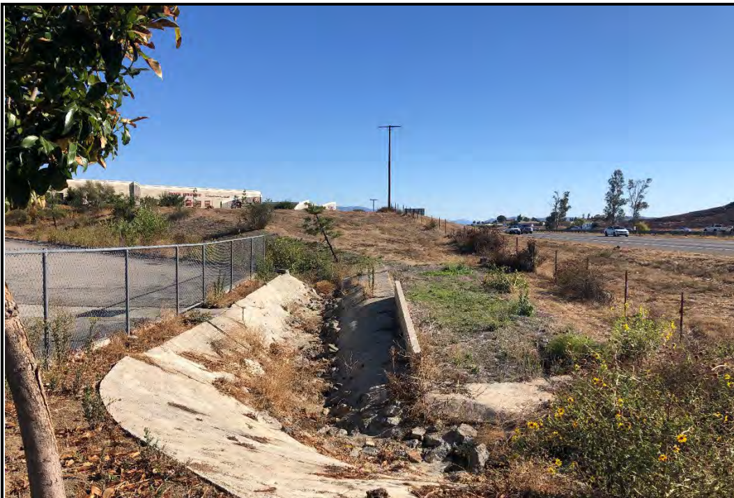
PHOTOGRAPH 4 View of Western Project Boundary at Stormwater Outlet, Looking Southeast
