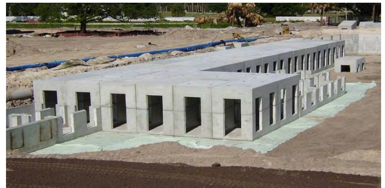
| StormCapture System During Installation Process
