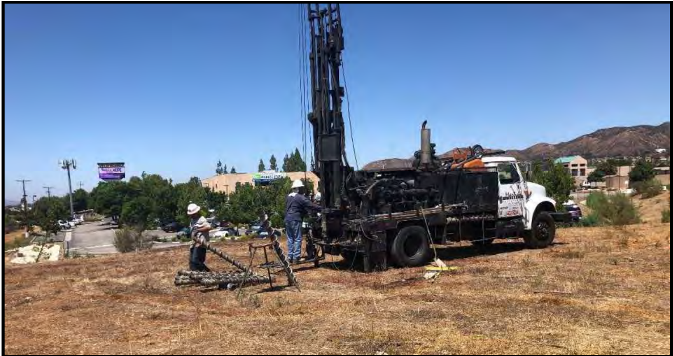
Figure 3-2. Geotechnical Test Boring B-1
