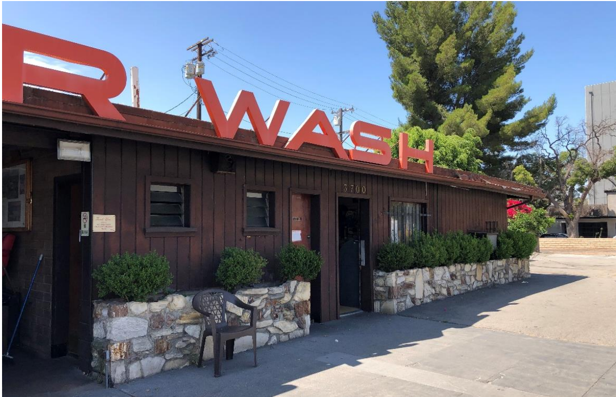
Figure 10 Main Bay, Facing Southwest
