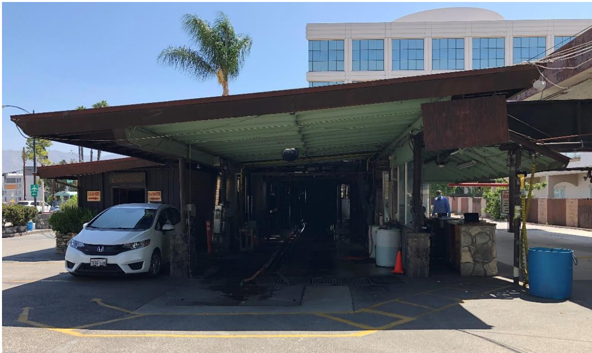
Figure 12 Main Bay and Car Wash, West Elevation, Facing East
