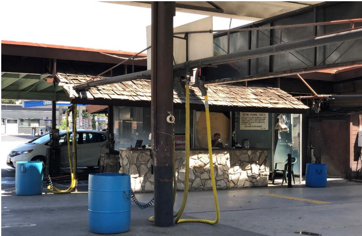
Figure 13 Cashier Kiosk, Main Bay, Facing Northwest
