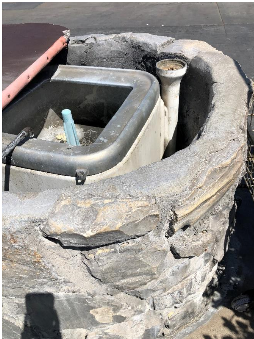
Figure 17 Rock Planter, Detail, Facing Northwest
