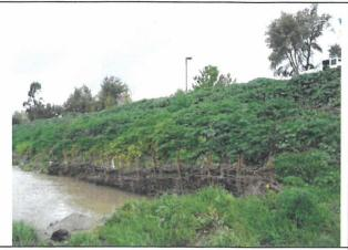
2) "Geoweb" (woven fabric cells) backfilled with native soils to repair eroded slope surfaces. In this example, after a brush wall was built the eroded areas were rebuilt with cellular confinement, then seeded and covered with erosion fabric, and seeded again. This low-impact method can be successful in some locations.
