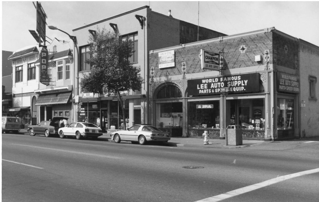
b) 1321-1323 Santa Clara Avenue (before 1897)
