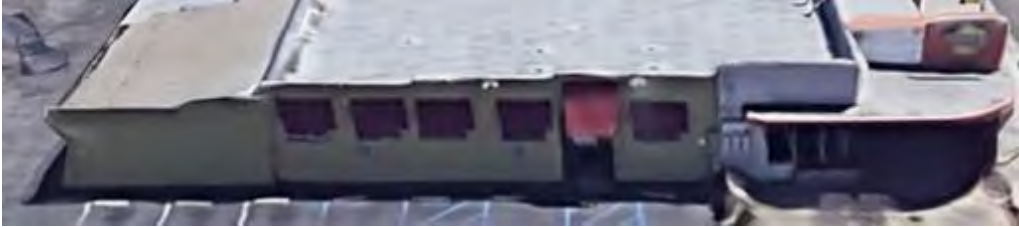
Photo of side (north) elevation of 126 N. Catalina Ave.
