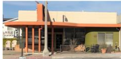
126 N. Catalina Ave., photo of front elevation
