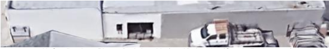
124 N. Catalina Ave., Photo of existing side (south) elevation (Google Earth, c2020)
