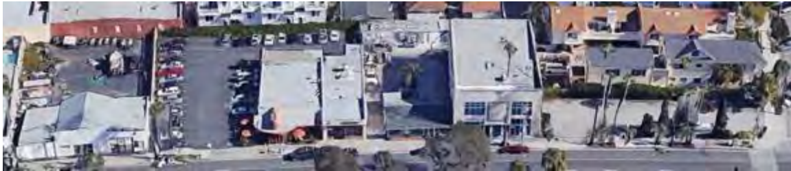
East side of the 100 block of N. Catalina Avenue (Google Earth, 2018)
