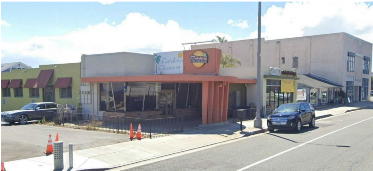
Figure 4 View of Commercial Use on Parcels along North Catalina Avenue, Looking Southeast
