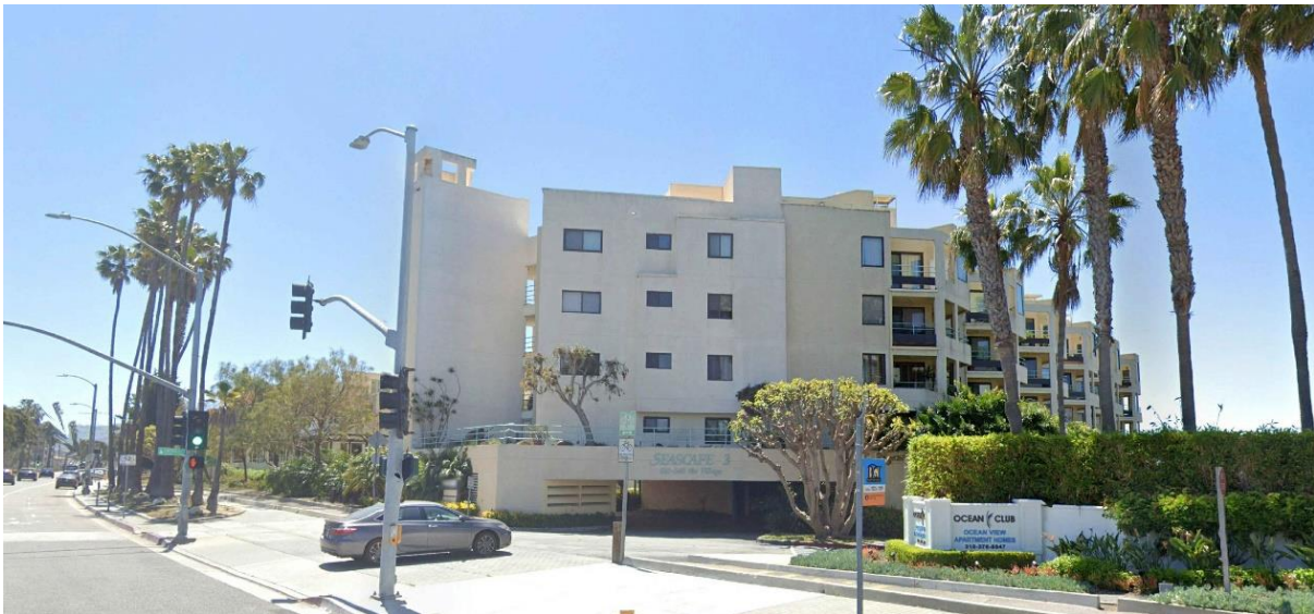
Figure 16 View of Existing Multi-family Residences south of the Intersection of Catalina Avenue and Emerald Street, Looking West
