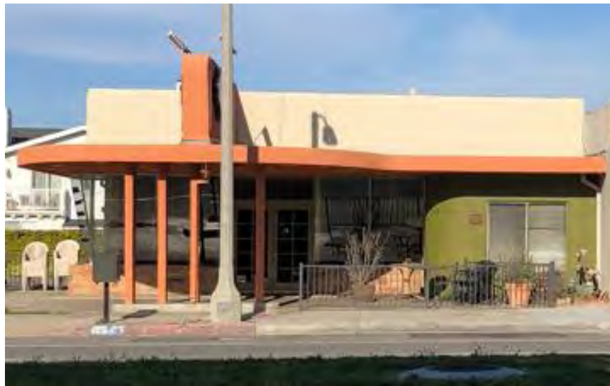
126 N. Catalina Avenue, west (front) elevation
