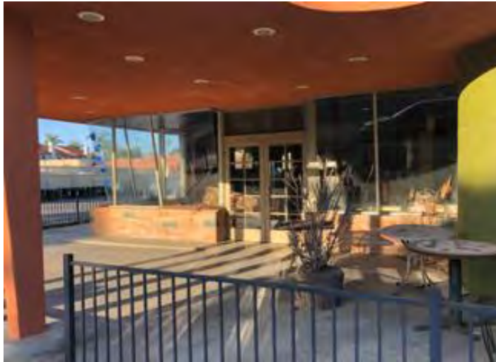
126 N. Catalina Avenue, west elevation
