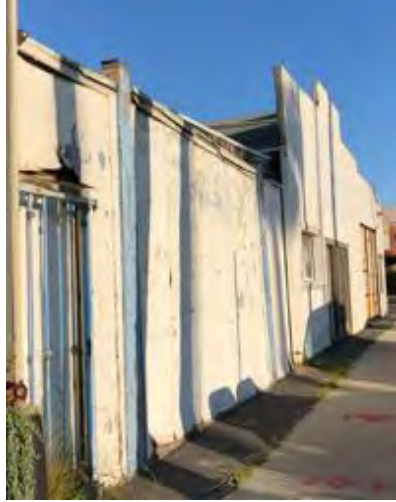
132 N. Catalina Avenue, west elevation
