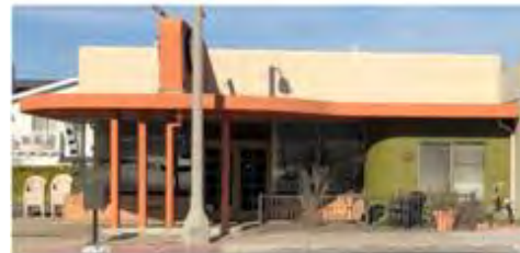
126 N. Catalina Ave., photo of front elevation
