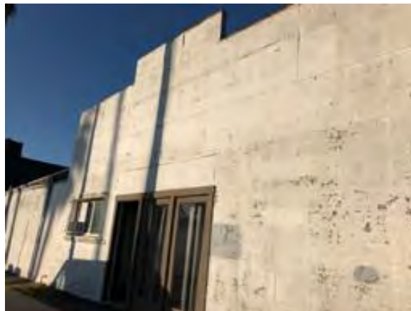
132 N. Catalina Avenue, west elevation
