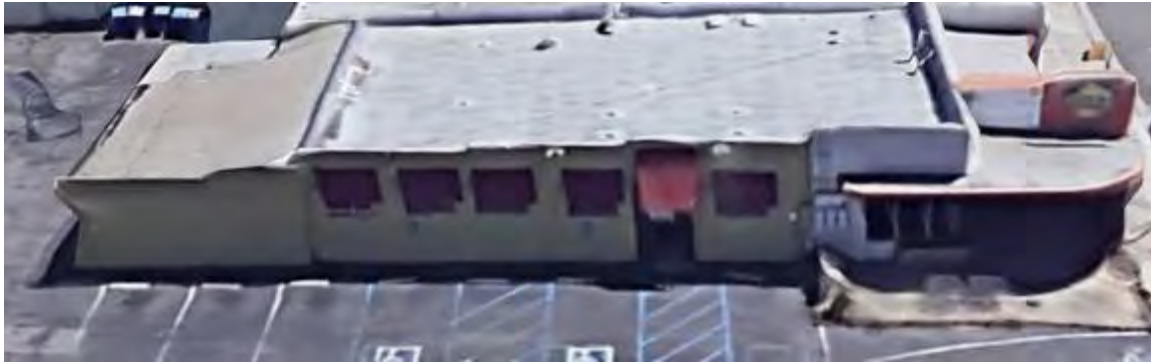
126 N. Catalina Avenue, north elevation (Google Earth, c2019)
