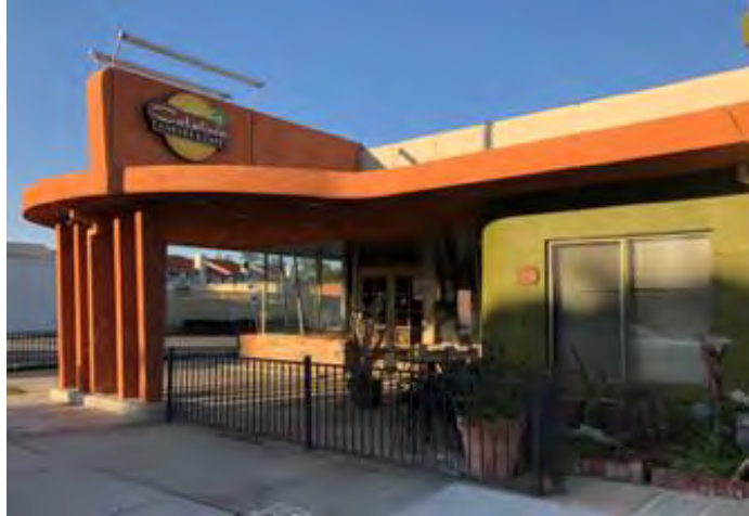
126 N. Catalina Avenue, west elevation and canopy
