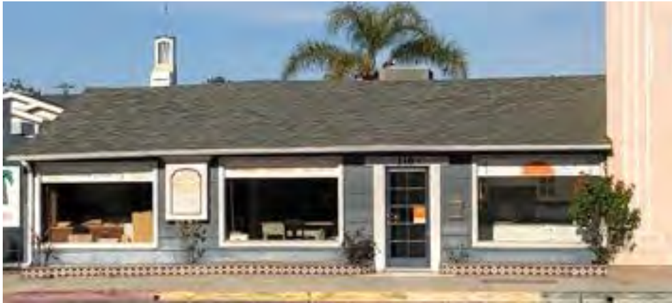
116 N. Catalina Avenue, front (west) elevation
