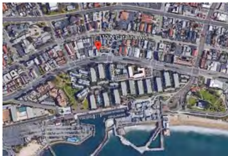
Area around 100 block of N. Catalina Avenue (Google Earth, 2018)
