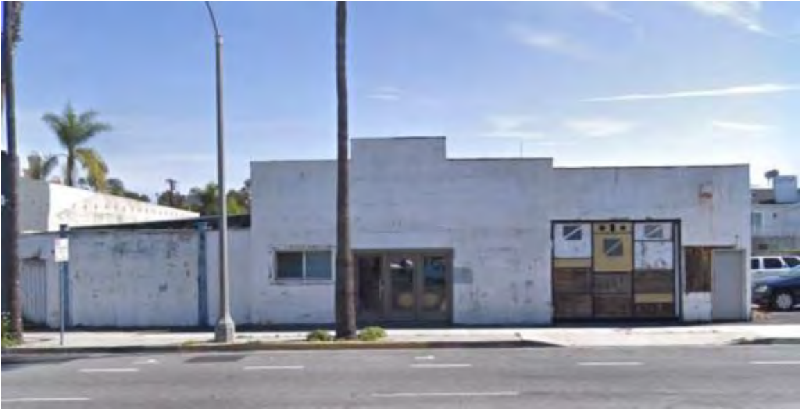
132 N. Catalina Avenue, west (front) elevation
