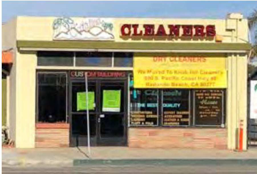
124 N. Catalina Avenue, west (front) elevation
