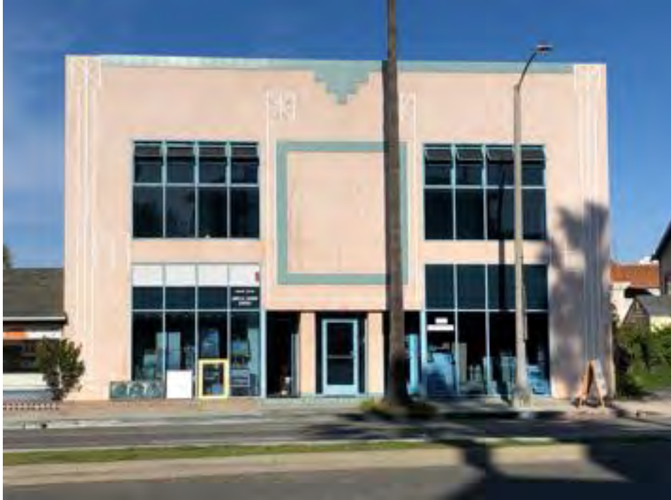
112 N. Catalina Avenue, front (west) elevation
