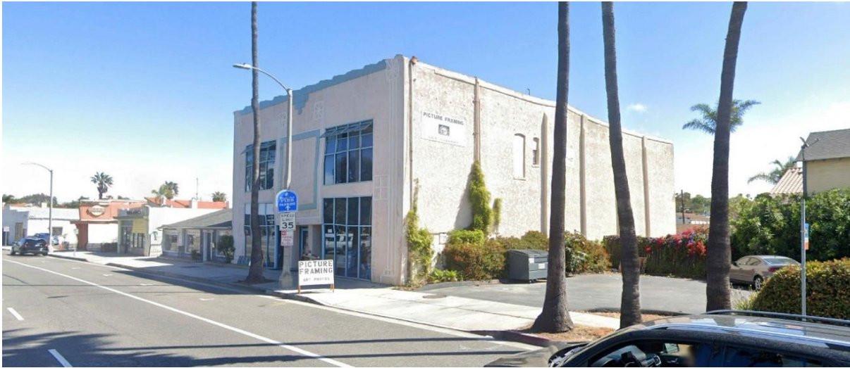
Figure 5 View of Existing Commercial Use on Parcels along North Catalina Avenue, Looking Northeast
