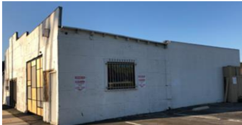
132 N. Catalina Avenue, front and side (south) elevations
