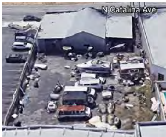
132 N. Catalina Avenue, rear (east) elevation and rear yard (Google Earth, c2019)
