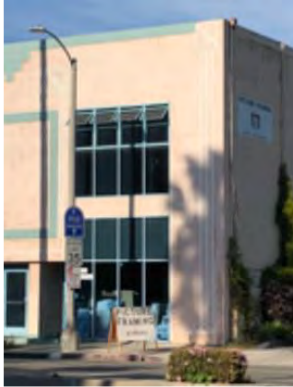
South end of west elevation, 2019
