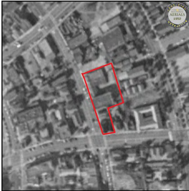
Figure 9. Project Area showing development (as depicted on 1952 aerial photograph)
