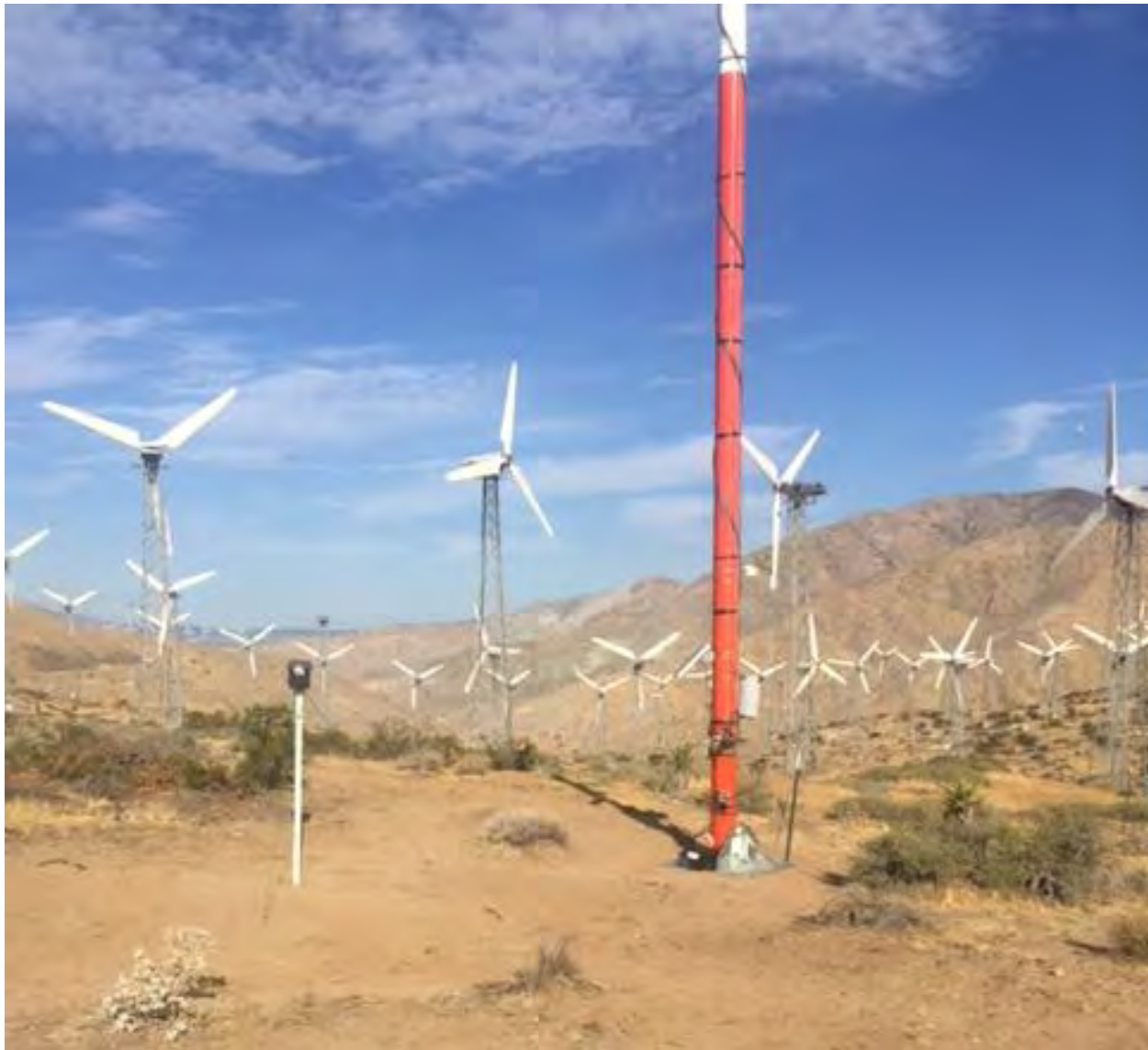
Figure 4. Acoustic sampling station at base of met tower showing near-ground detector mounted on 1.5-meter pole and base unit mounted to elevated microphone.
