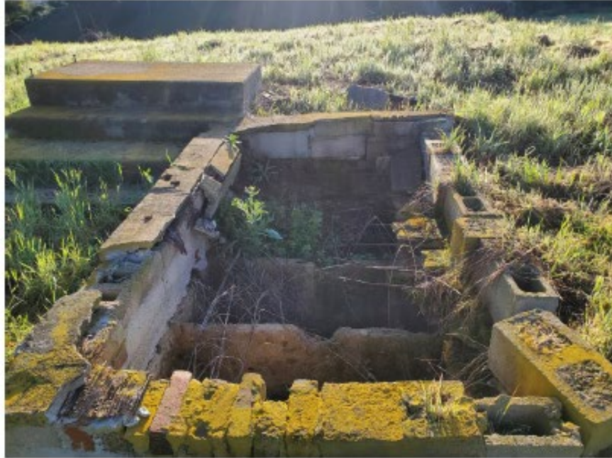
Photograph #7 Concrete foundation debris in central-eastern portion of the Site.
