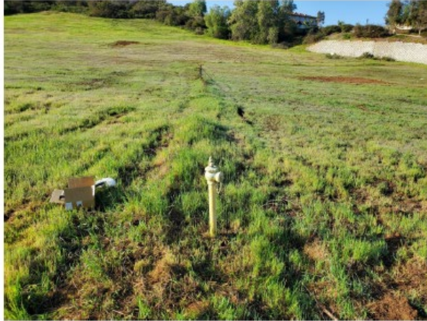
Photograph #11 Water line located in the central-northern portion of the Site.
