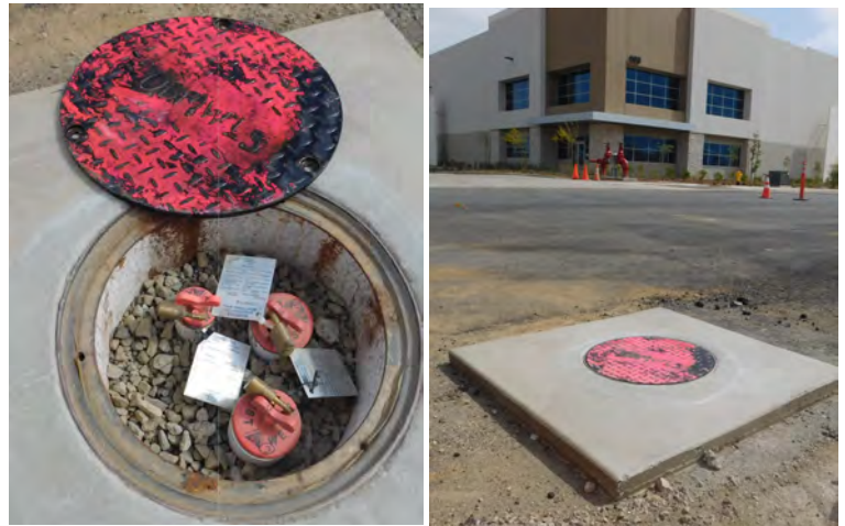
Off base PFAS monitoring well being modified for street upgrade
