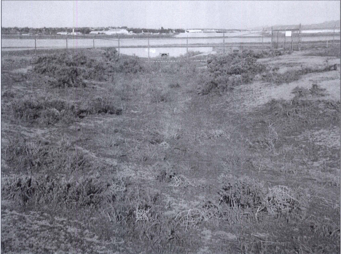
Figure 1. Northwestern portion of the flood control channel where it drains from a concrete pipe culvert located along the south side of a taxiway on March ARB (view to the north-northwest). From here, it drains southeasterly across the property and into a modern, concrete pipe culvert.
