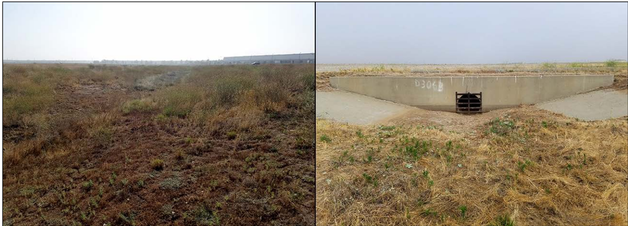
Site 33-024853 in 2020. Left: overview to the southeast; right: culvert under Taxiway A (Feature 1), view to the northwest. (Photographs taken on June 23, 2020)
