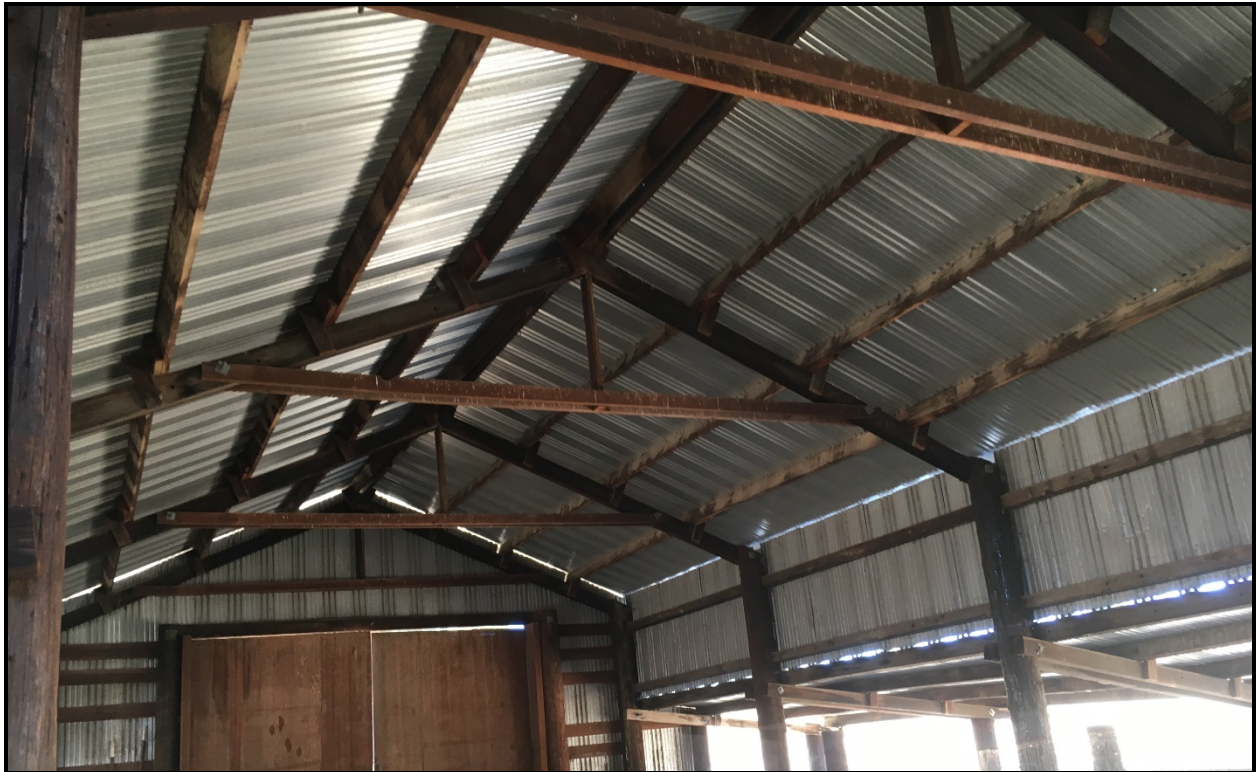
Photo 7. View of barn planned for removal. Photo taken 9/20/19.
