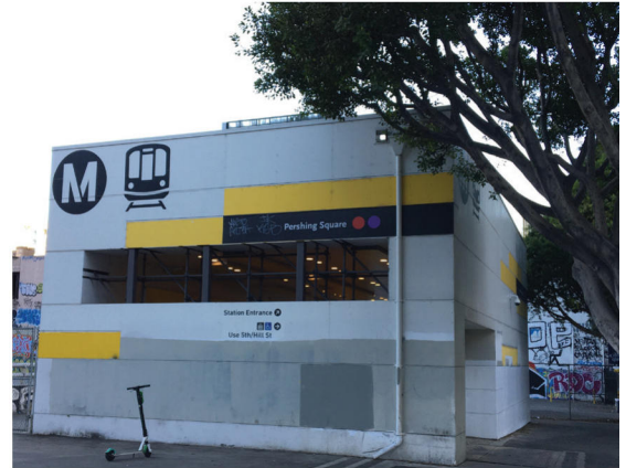
Constructed above is a wooden box over the entrance portal for overhead protection at the 4th/Hill Station.
