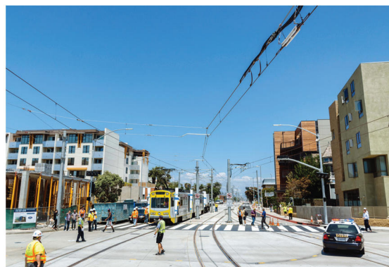
Trained flaggers ensure the safe crossing of pedestrians and workers of an adjacent development.
