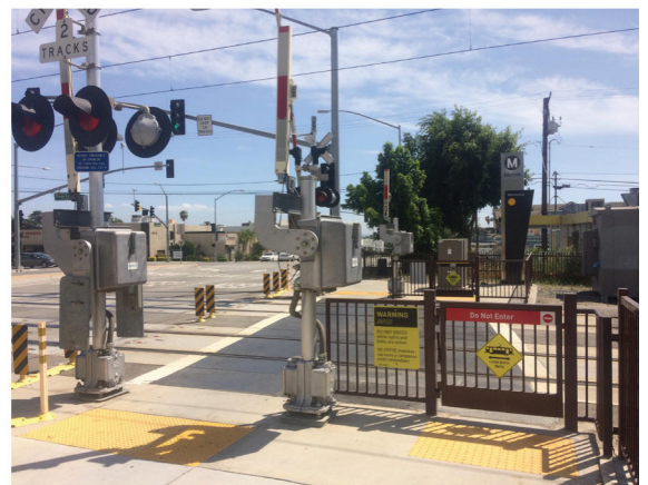
Safety elements of a gate and pedestrian arms have been constructed at the Monrovia Station.
