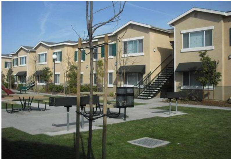
FIGURE 4.10-5: KENDREA PLACE APARTMENTS IN NORTH MCFARLAND, ALONG ELMO HIGHWAY
