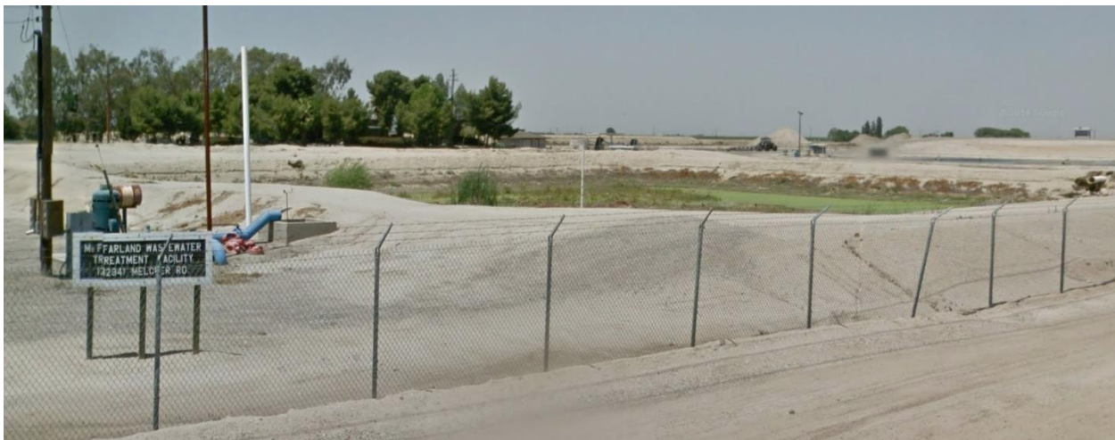
FIGURE 4.10-8: MCFARLAND WASTEWATER TREATMENT PLANT, ALONG MELCHER ROAD
