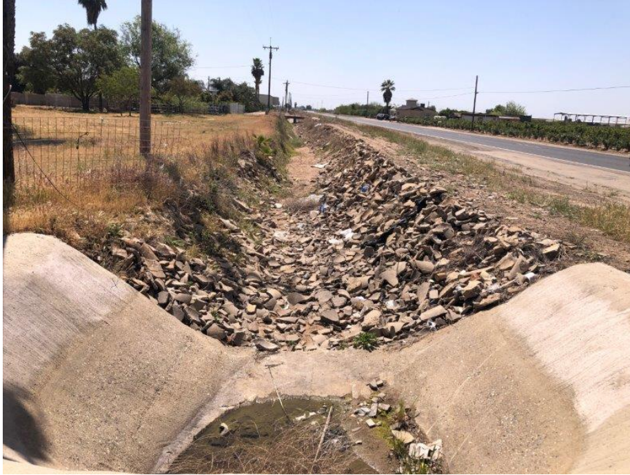
Photo 15 (above). Tout Ditch along Road 120 in Orosi.
