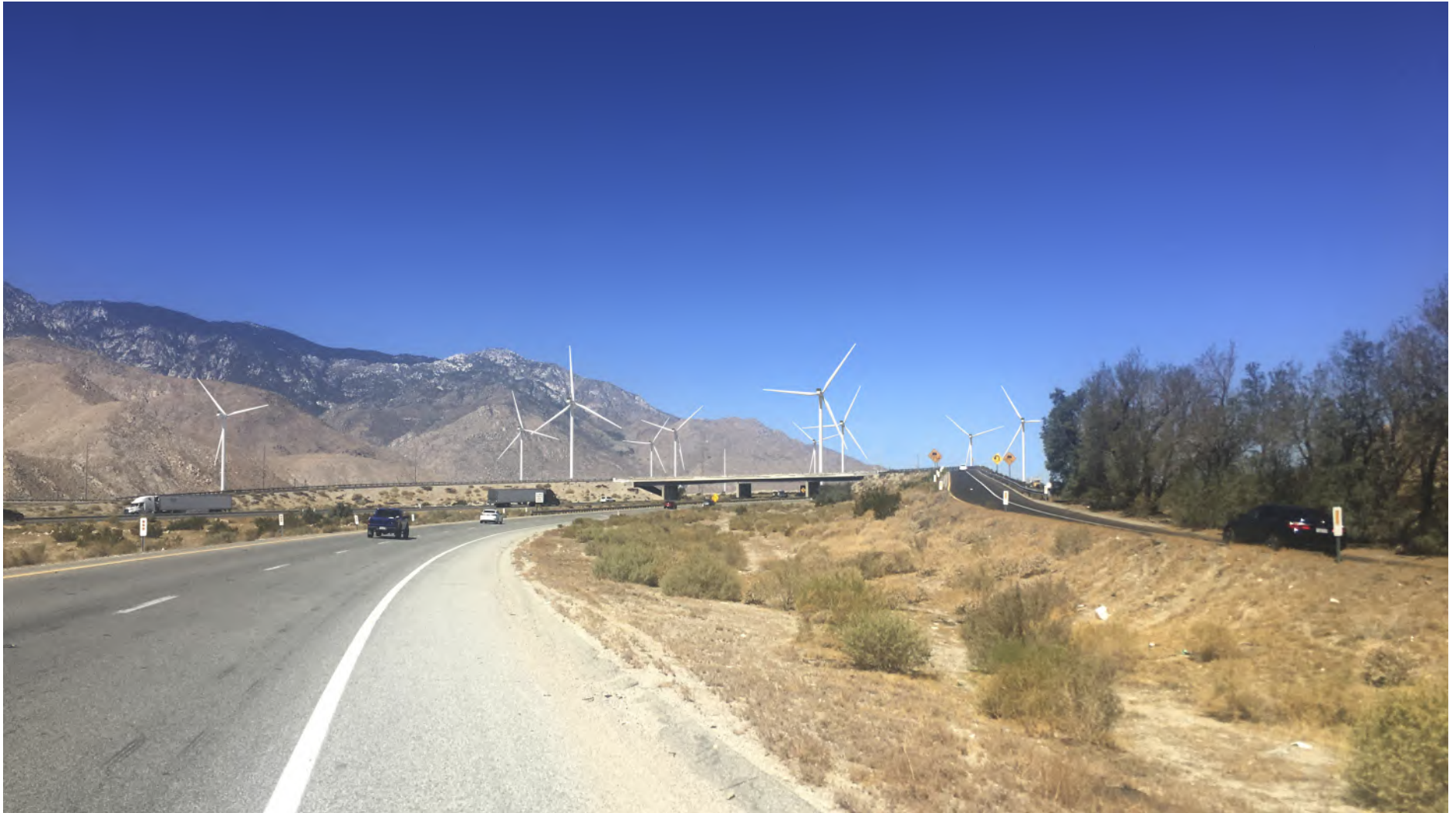
View southeast from southbound SR-62 towards Project Site (proposed conditions)
