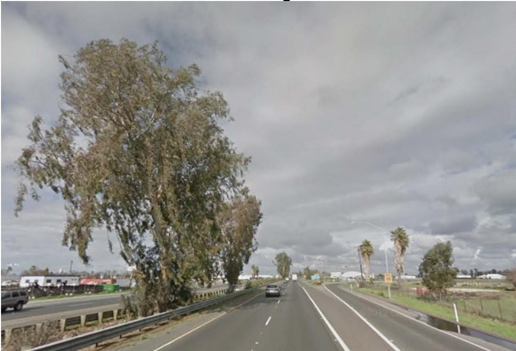
Figure 2-3: Existing Conditions of State Route 99 at Post Mile 25.4, North of the Avenue 200 Overcrossing
