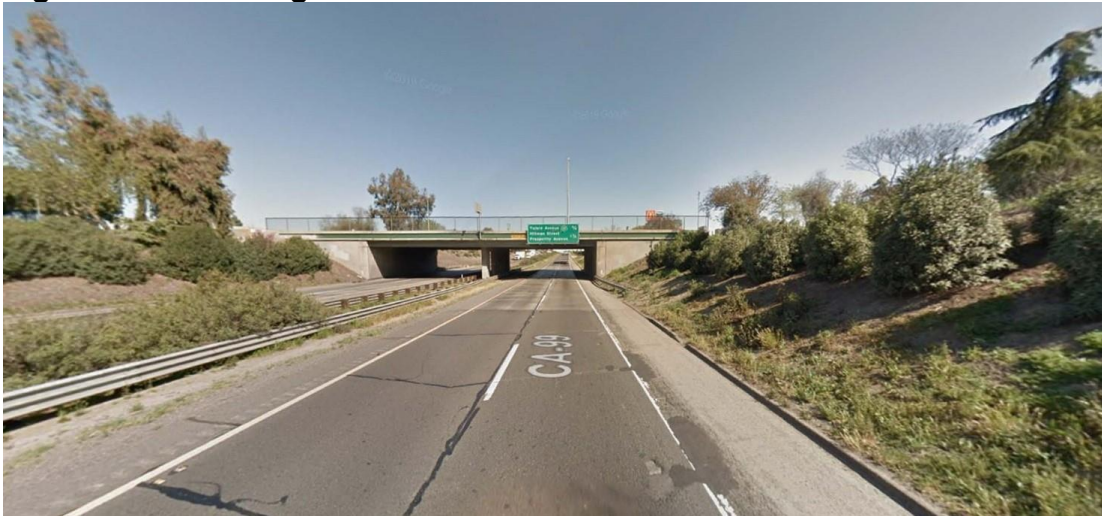
Figure 2-7: Existing Conditions at Post Mile 28.5
