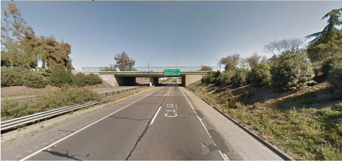
Figure 2-7: Existing Conditions at Post Mile 28.5
