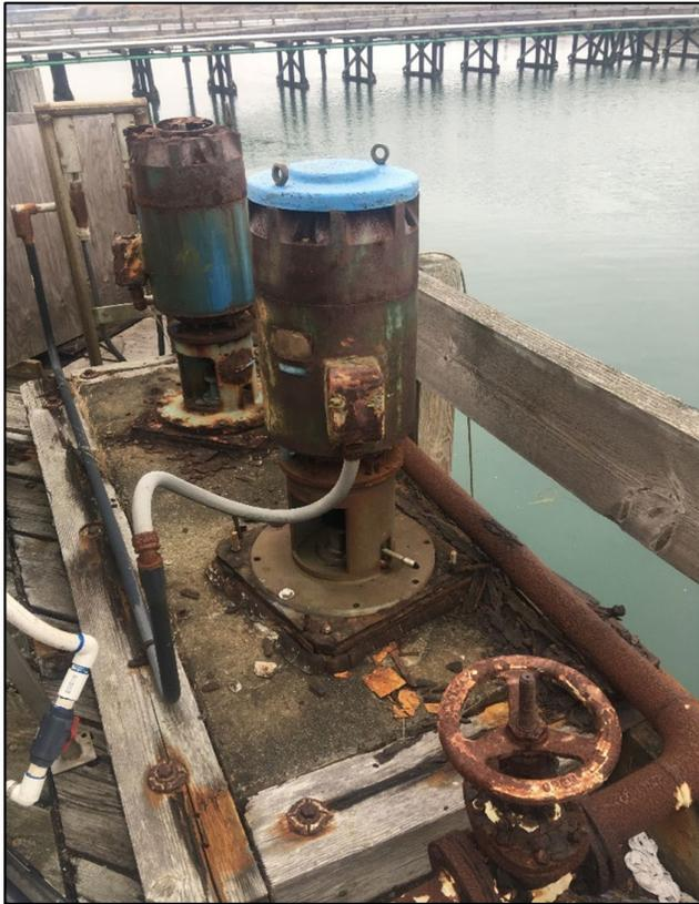
*Image 2-14 RMT II-Existing Water Intake Pumps*
