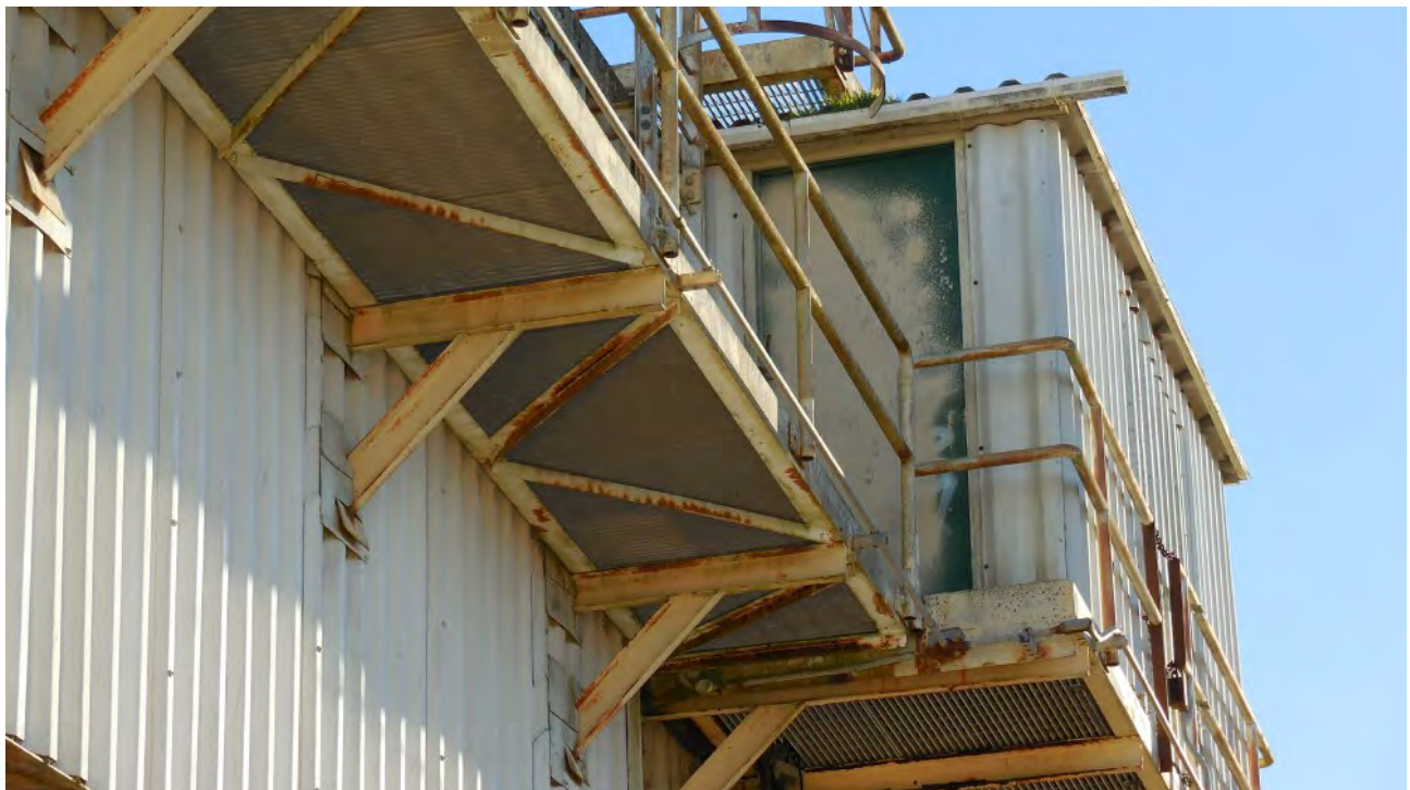
Figure 22. No signs of past or present bat activity in connected structure.
