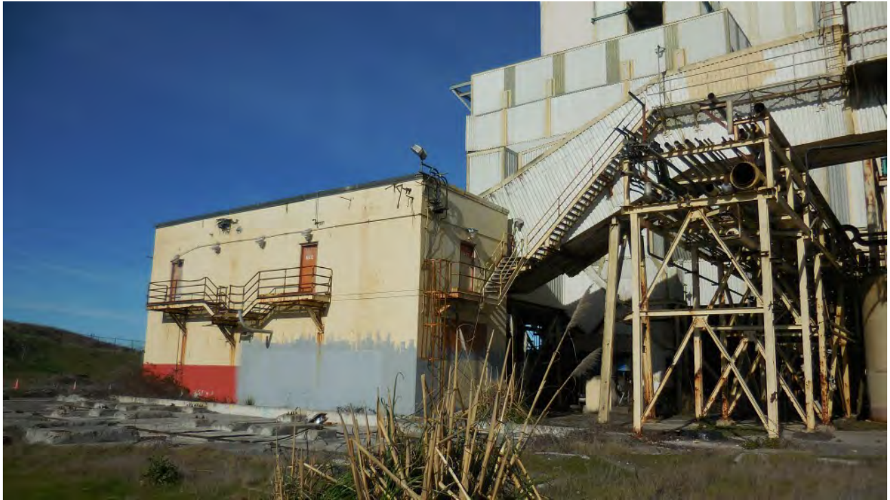
Figure 23. 2-Story Building near Smokestack and 12-Story Boiler Building. No signs of use by bats around exterior or interior.
