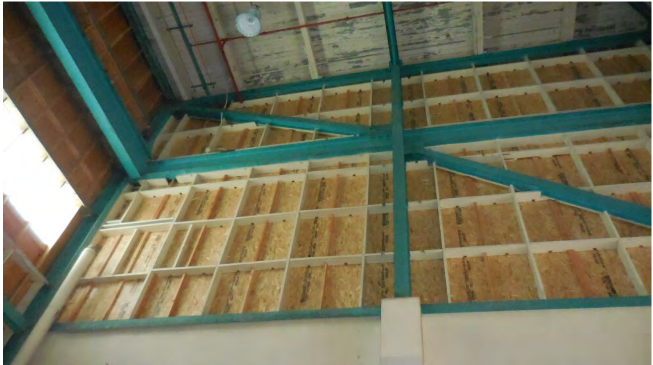
Figure 44. Wall at entry to Warehouse and Shared Spaces.
