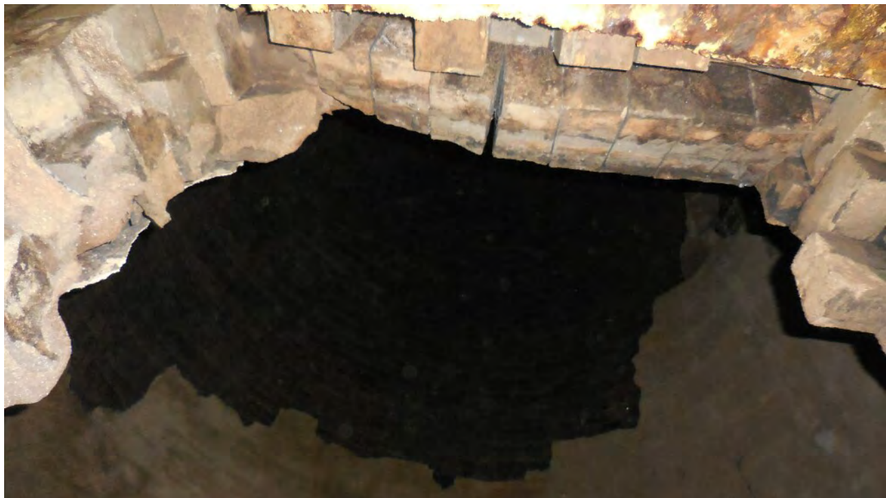
Figure 26. Interior lower portion of Smokestack. No signs of roosting bats.
