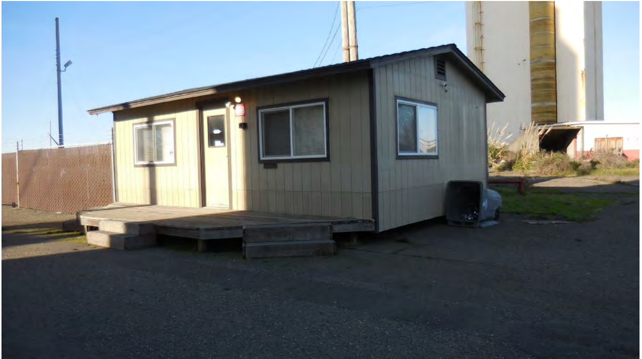
Figure 40. Portable building outside north boundary – no signs of use by bats, no suitable entry points.
