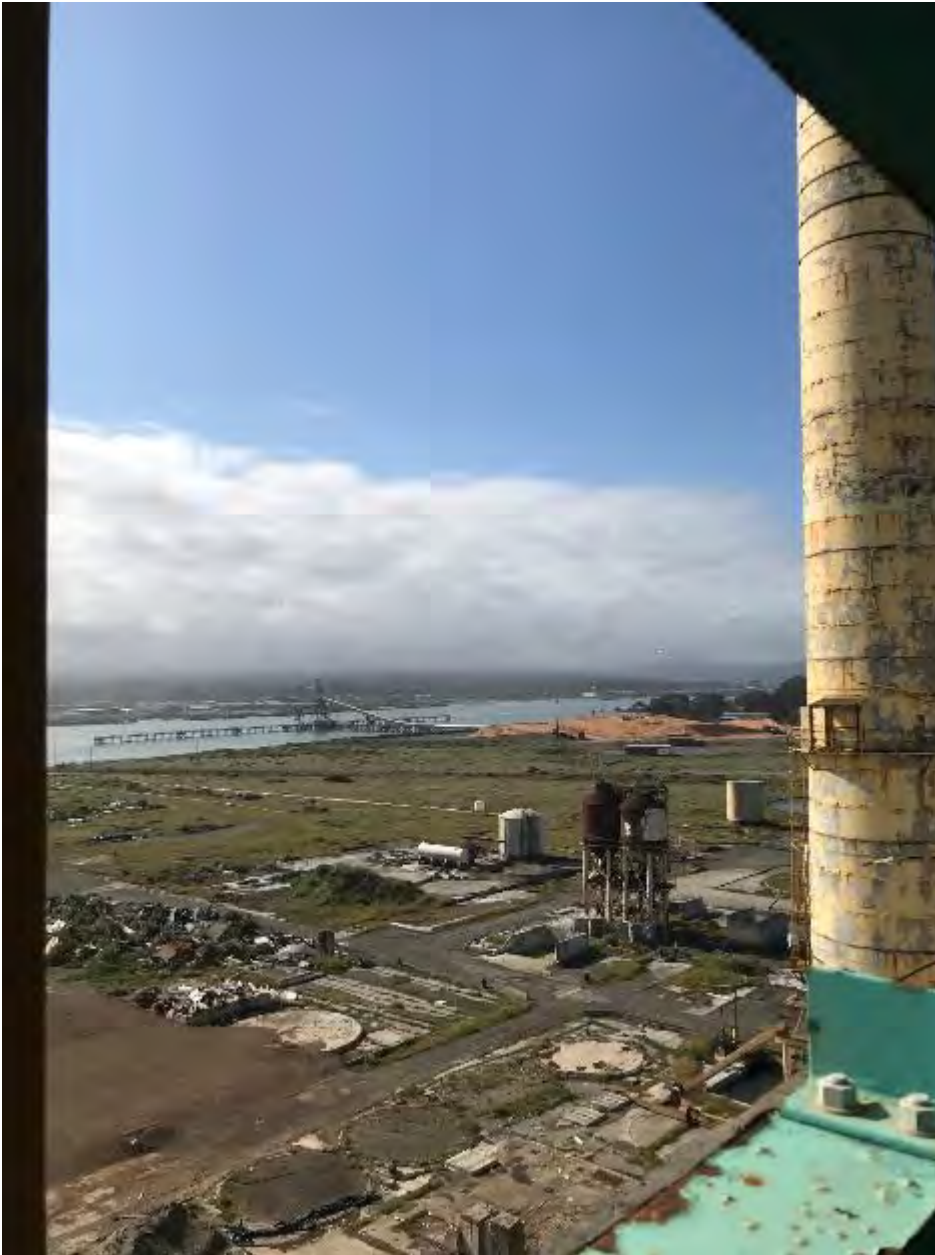
Photo 17. View of Project Site from mid-level window of main boiler building with view of Humboldt Bay channel in the distance.
