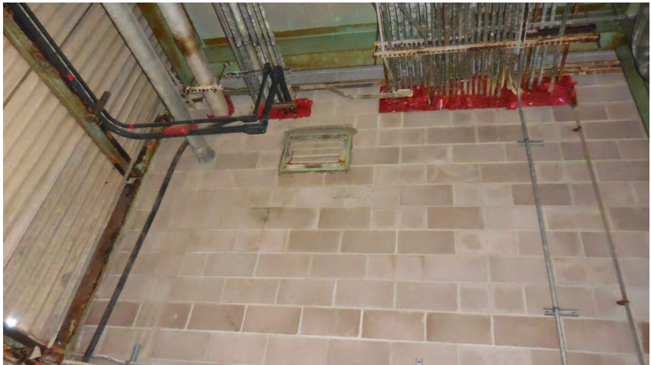
Figure 33. Interior, 3-Story Boiler Building.
