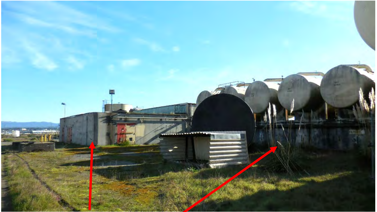
Figure 11. Filter/Softener Tank Building (left) and attached Tank Support Building (right)
