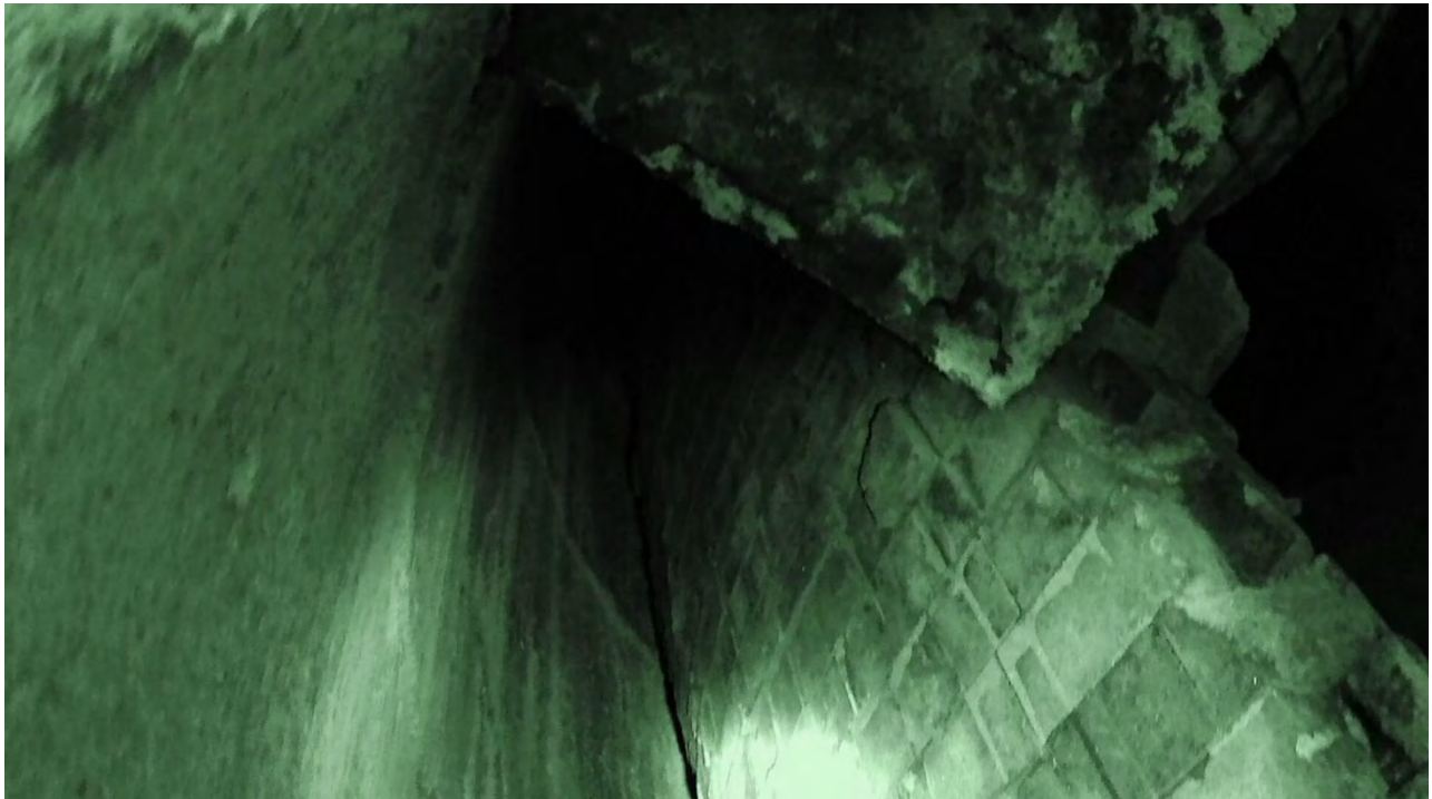
Figure 28. South-facing portion of 3-Story Boiler Building just east of 12-Story Boiler Building. No signs of bat activity, exterior or interior.
