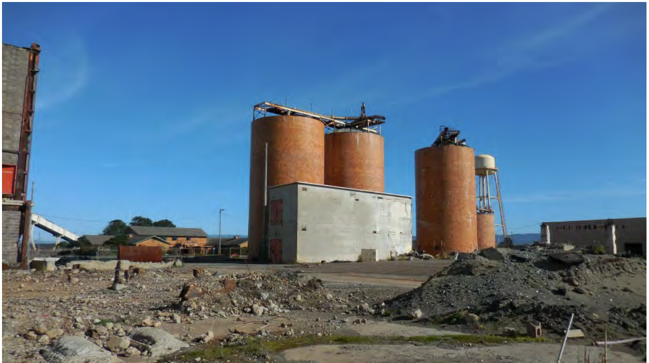
Figure 35. Brick Silos (tanks) located at north-central portion of site. Structure 2 is visible in foreground. No signs of past or present use by bats in Structure 2, tanks not safe to survey interiors, but 2 have open tops, no suitable habitat; remainder have no suitable openings for bats.
