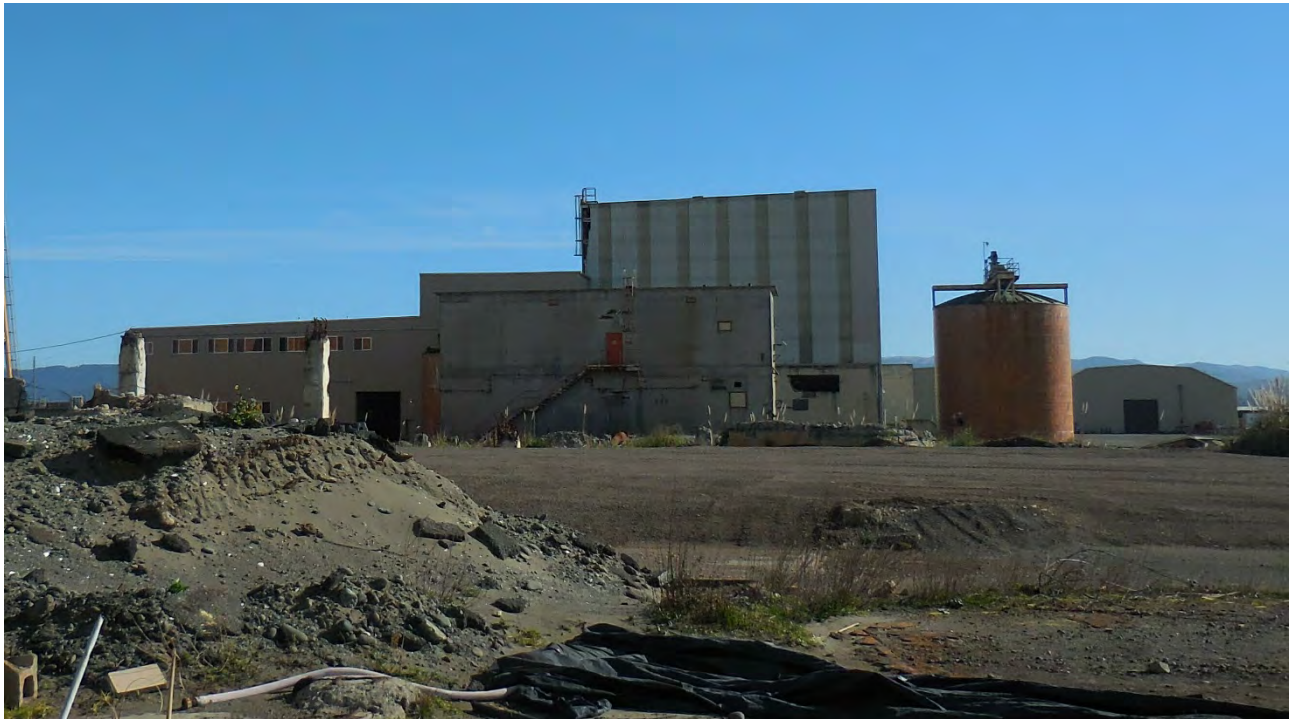
Figure 41. Structure – 2-story building in foreground, Existing offices at left side of large structure, Warehouse and Shared Spaces in central part of building behind Structure, and Machine Building and Silo at right.
