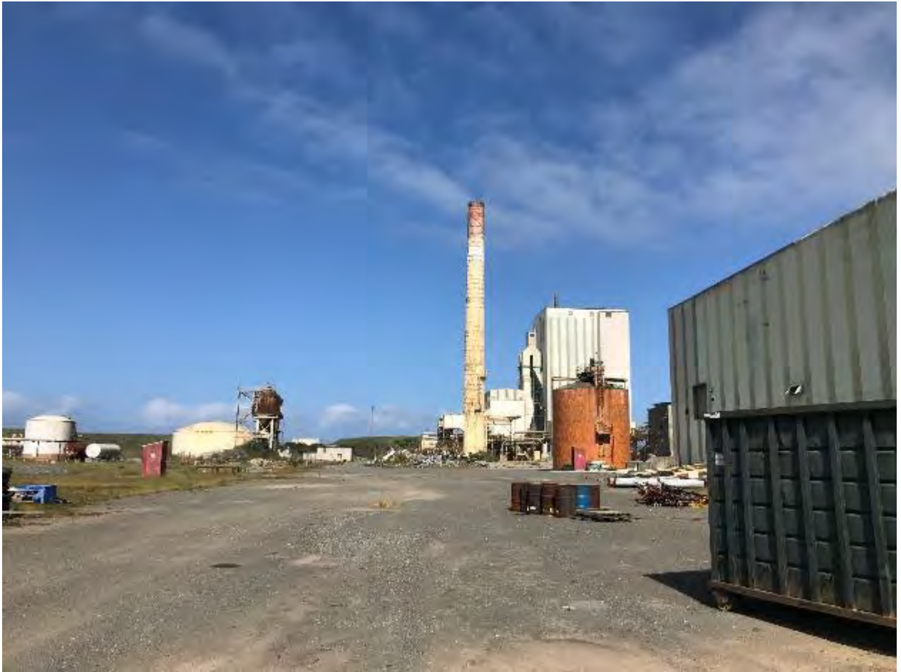
Photo 16. View of buildings on-site with large warehouse to the far right, and the main boiler building center-right.
