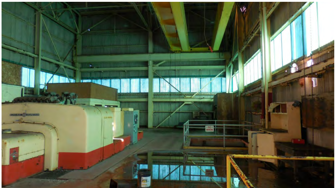
Figure 34. Interior, 3-Story Boiler Building.
