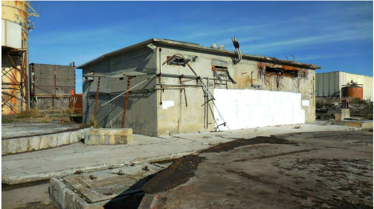
Figure 7. Building SUB FL.2. Bat activity noted in several interior locations.
