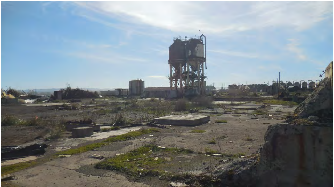
Figure 37. Steel tanks in interior of site. No suitable bat habitat.
