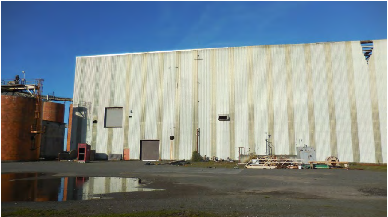
Figure 51. Continued view of Machine Building. Extremely large structure has many large openings in walls and roof. No signs of past or present use by bats observed around exterior, or in interior large open spaces or enclosed rooms.
