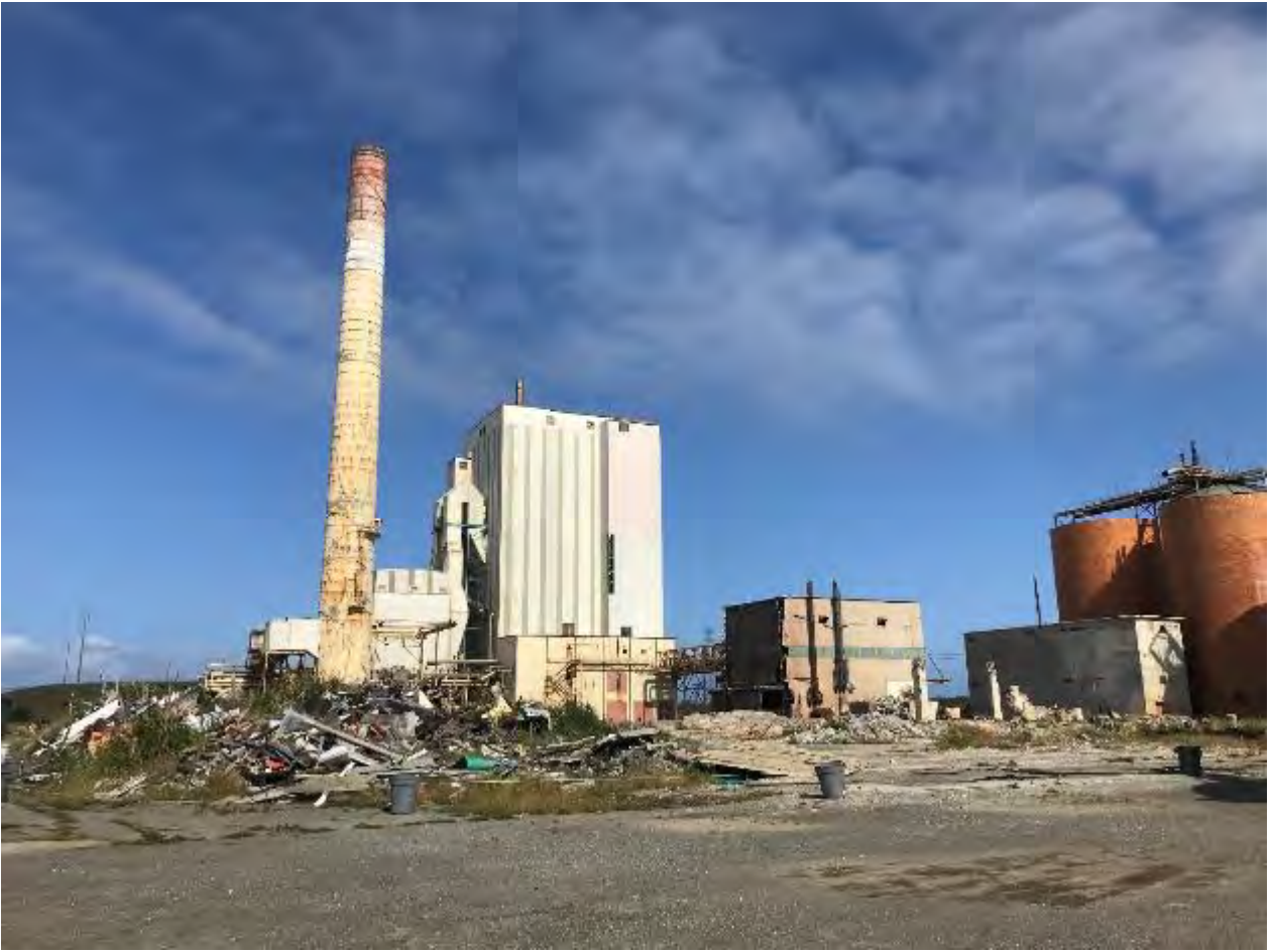
Photo 13. View of buildings and demolished materials on-site (facing west).
