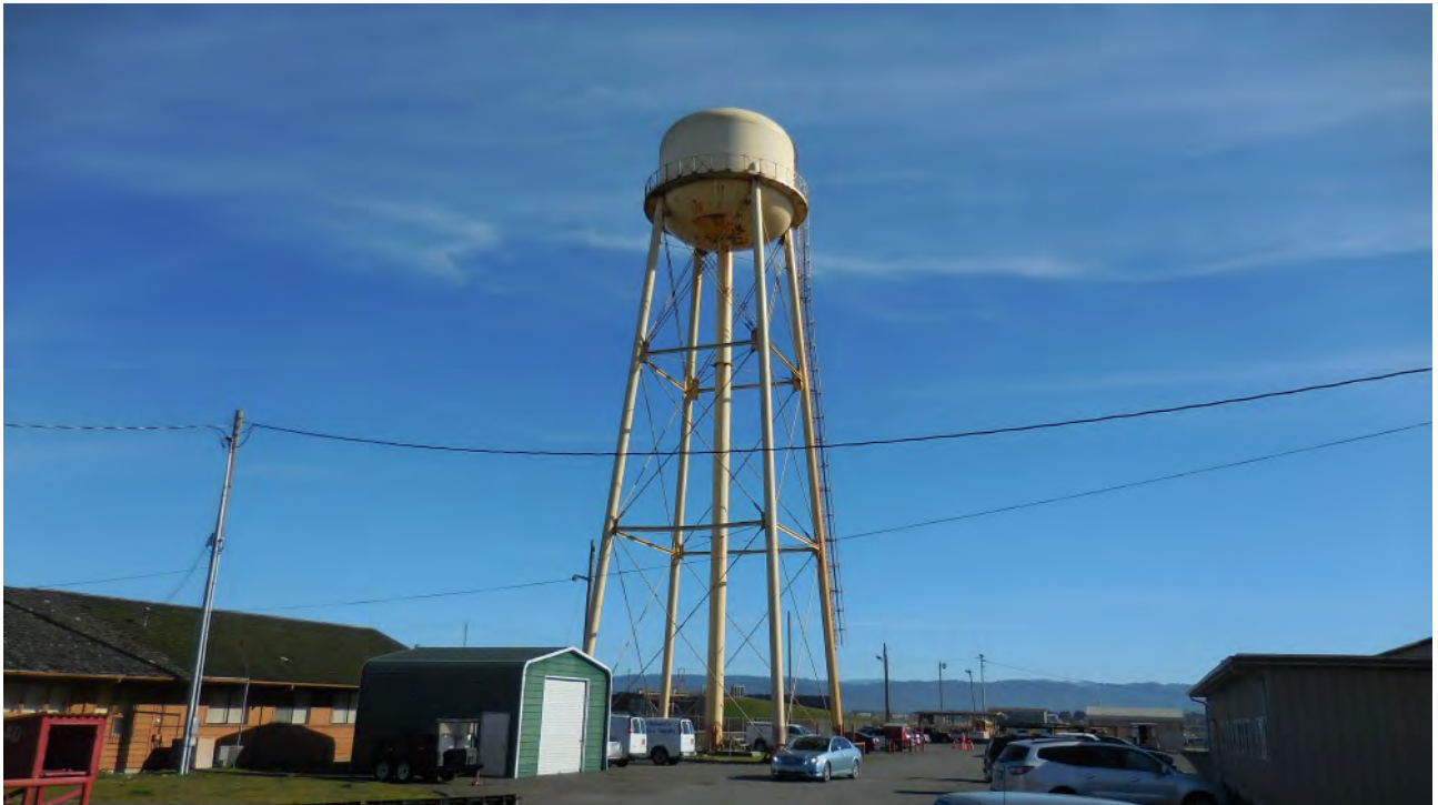
Figure 38. Elevated water tank, north portion of site just outside boundary, but may be removed. No suitable bat habitat.
