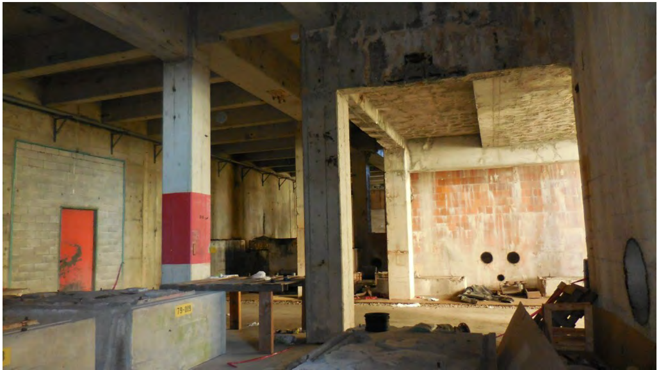
Figure 55. Interior of Machine Building – large amounts of light and airflow, not conducive to bat roosting activity, even in more protected locations such as this concrete wall and girder ceiling area.
