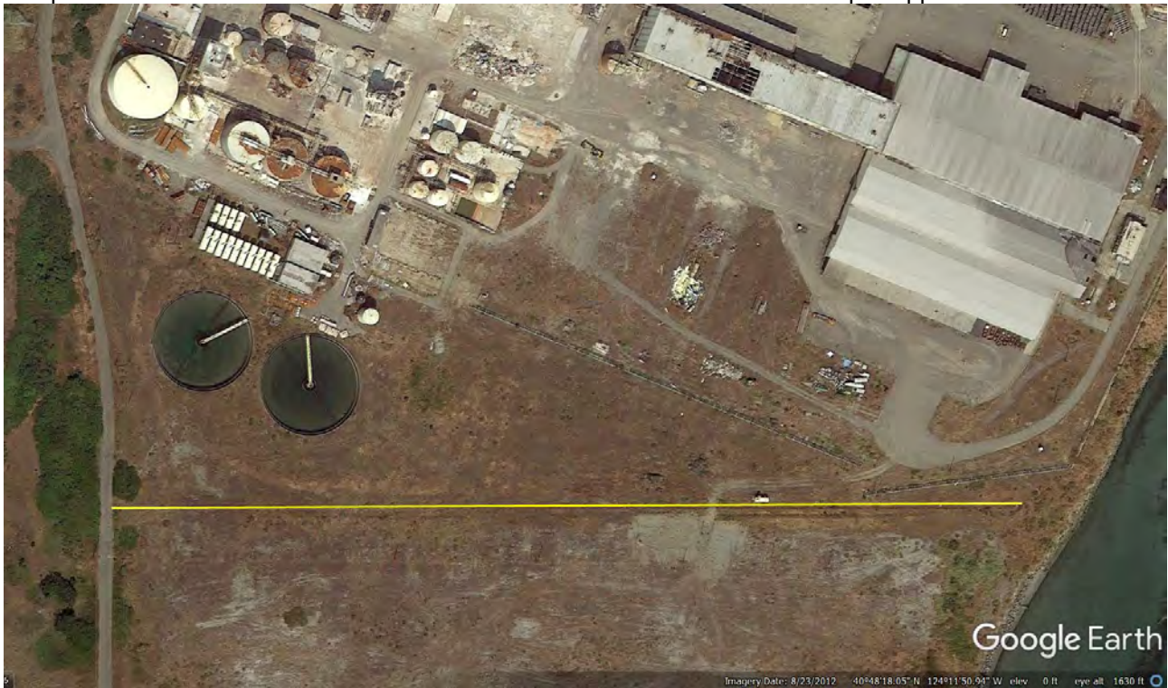
Figure 10. Imagery from 2012 shows grading around the fence gate between the sand berms and the current locations of railroad tie debris piles.
