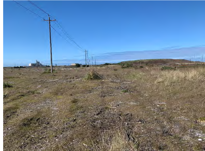
Photo 15. Grading and dredge debris south of the sand berm.
