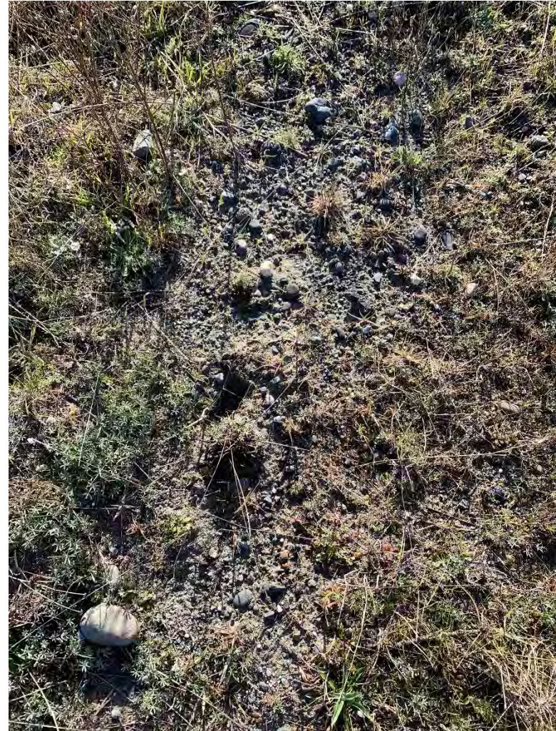
Photo 2. Scattered gravel in degraded dune mat near the clarifiers.
