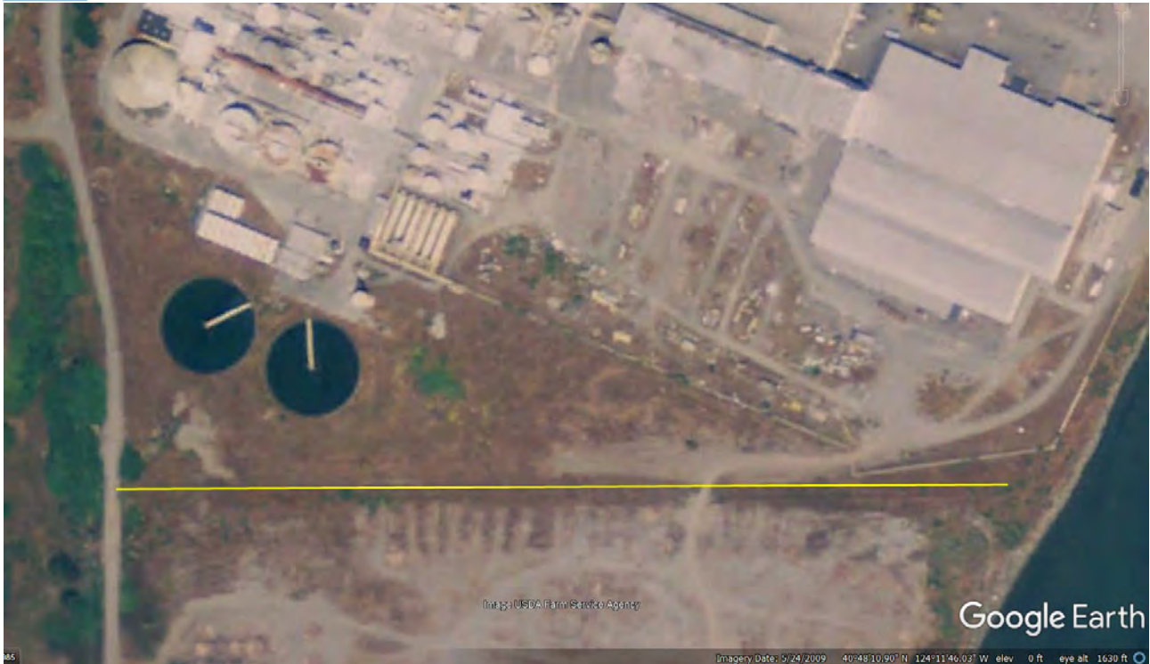
Figure 9. Imagery from 2009 shows additional grading and disturbance on both sides of the southern fence line and pit near the clarifiers. The former rail lines are removed and the first debris pile appears.
