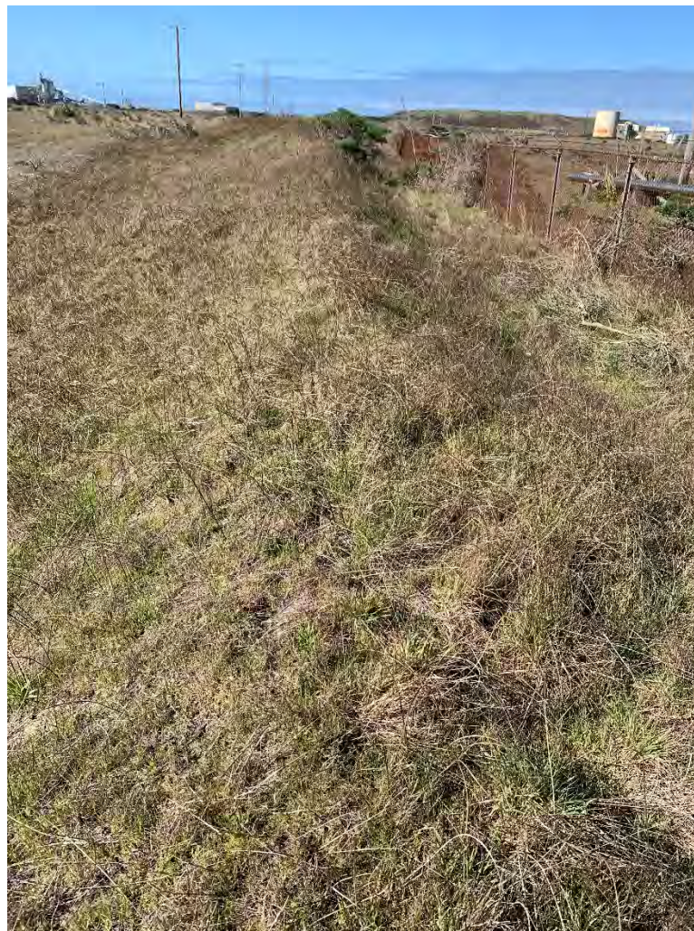
Photo 12. Stabilized eastern sand berm south of cyclone fence.
