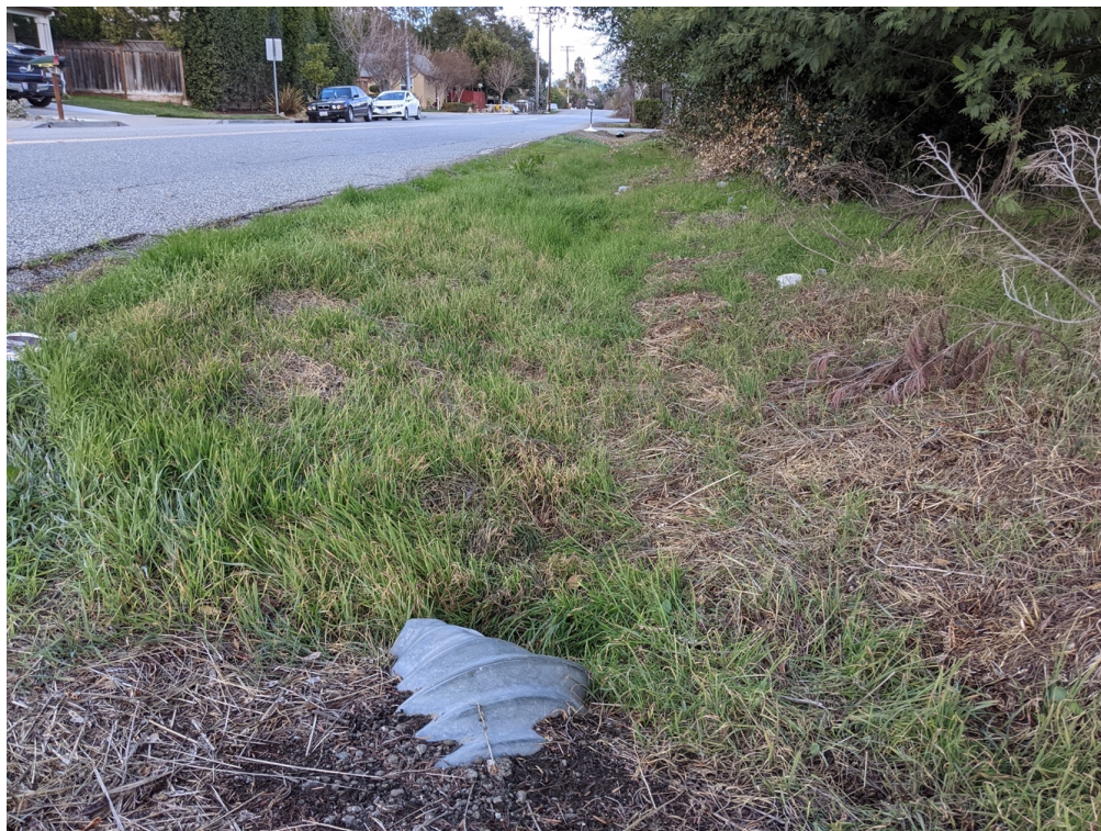
Photo B-2: Culvert along Kern Avenue. Photo taken facing N.
