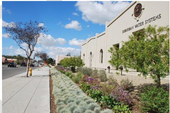
One of the Public Water Utility Companies in Whittier
