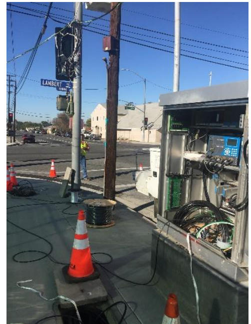
Traffic signal maintenance along Lambert Road
