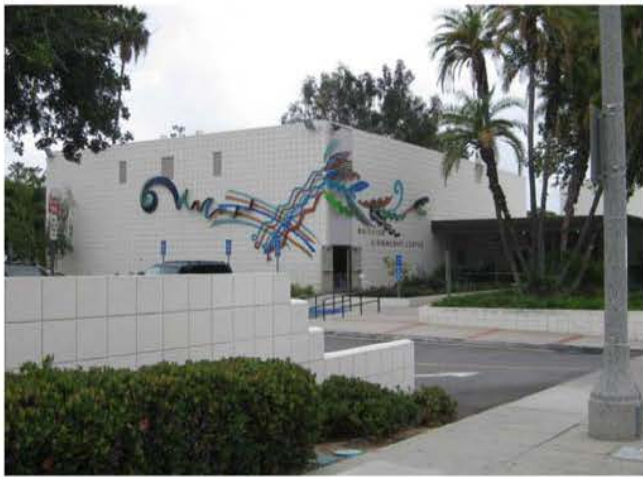
Whittier Community Center Envision Whittier Existing Conditions Atlas
