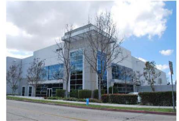
A warehouse along Whittier Boulevard
