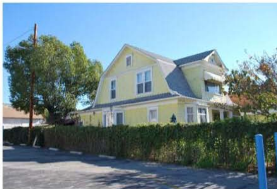
Older residential building in Uptown
