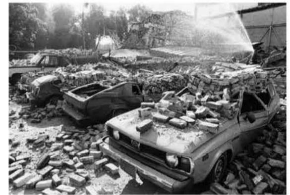
Masonry damage from 1987 Whittier Narrows Earthquake
