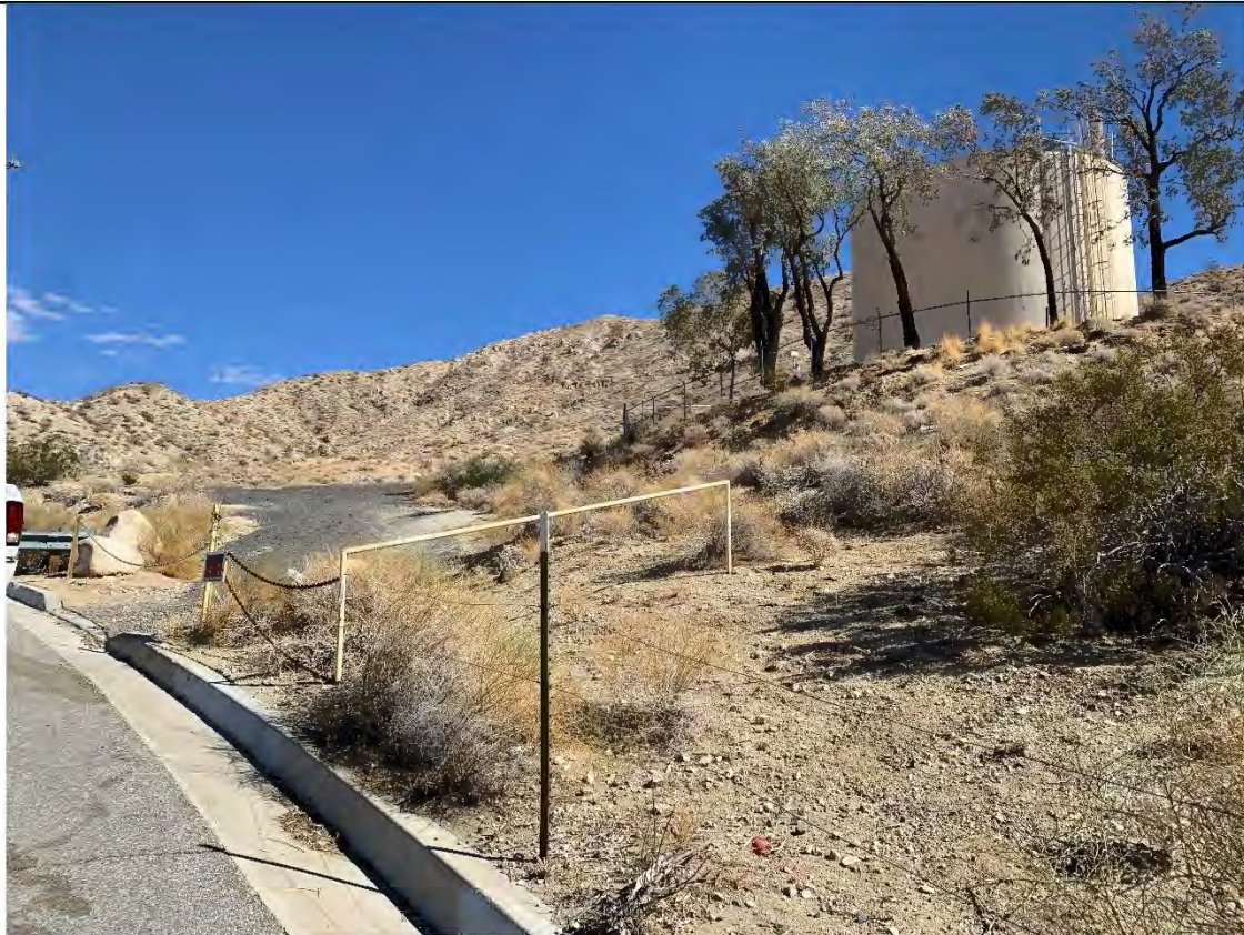
Photo 1. Looking north at the existing reservoir and access road.
