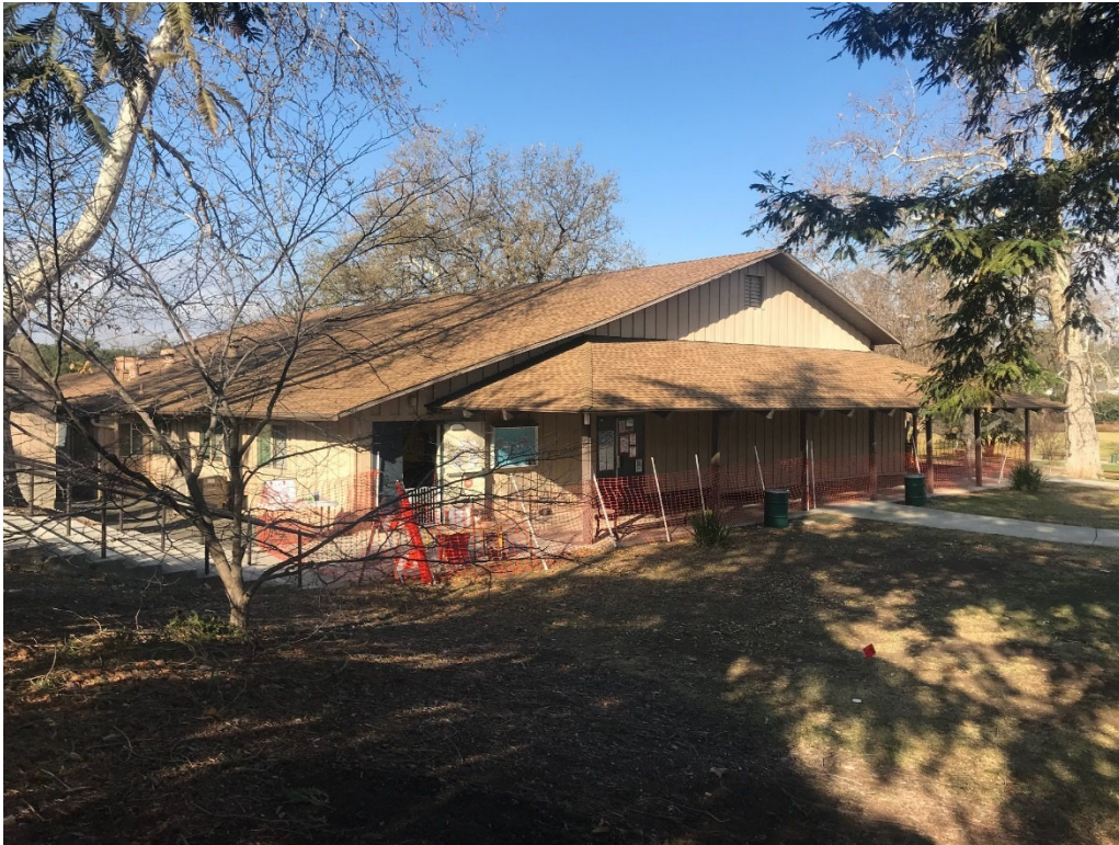
Figure 19 Community Center Building, Facing Northwest
