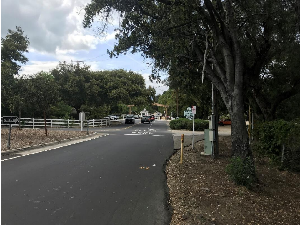
Photograph 5: Overview of western portion of the project site. Photo facing northwest along Long Valley Road.
