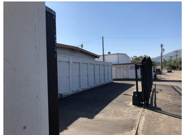
Photo #10 View of Stow-It Self Storage (215 South Bent Street) located to the adjoining south of the site.
