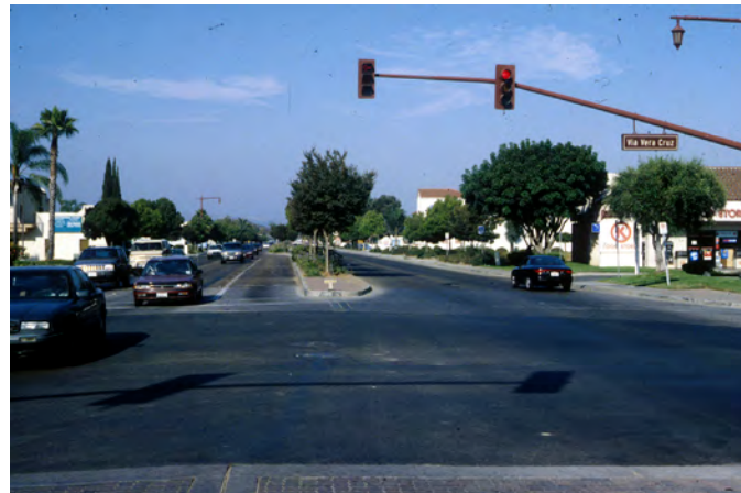
San Marcos Boulevard is a heavily traveled commercial corridor and sub-regional thoroughfare.
