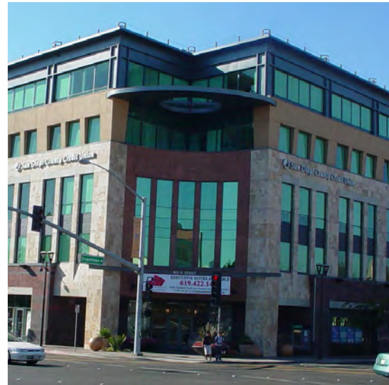
At street corners, the street wall may be set back diagonally to emphasize the intersection and to extend the public realm.
