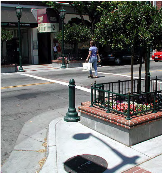
Bollards should be used to demarcate and protect pedestrian areas.
