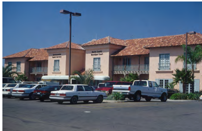
A nearby office building reflects a Spanish/Mediterranean style.
