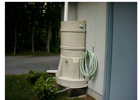
District development should incorporate water conservation features including drought-resistant landscaping (top), low-flow fixtures (middle), and rainwater harvesting (bottom).
