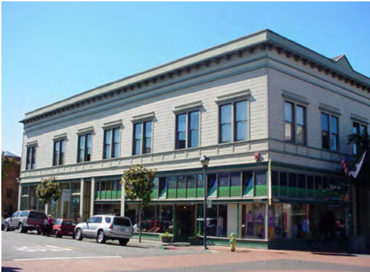
Commercial buildings should be simple in form and massing; this building has a storefront base and a detailed parapet
