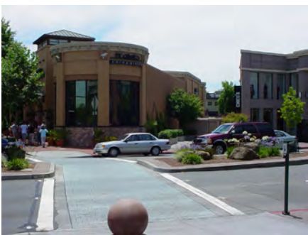
Special paving treatments draw drivers' attention to pedestrian crossings while adding aesthetically to the pedestrian environment.
