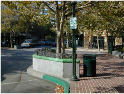
Curb extensions slow traffic, reduce pedestrian crossing distances and expand the pedestrian realm.
