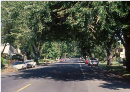
Bent Avenue will have parking and bike lanes on both sides
