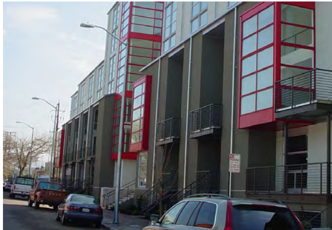
A variety of housing types, including “live-work” units, will establish a diverse residential community and provide for flexibility in the area's redevelopment.
