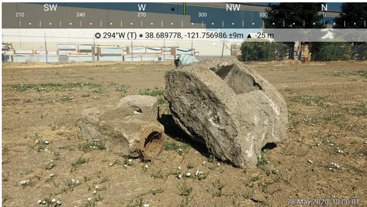
Photo 10: An example of concrete debris from former storm drain infrastructure present within the western side of the Project site, looking west.
