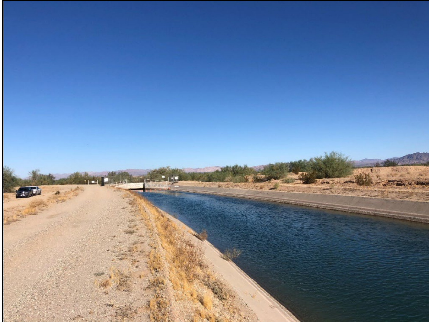
Photo 3. Section of the Coachella Canal within the northwestern portion of Study Area 2, between project impact areas; photo facing northwest. November 9, 2020.
