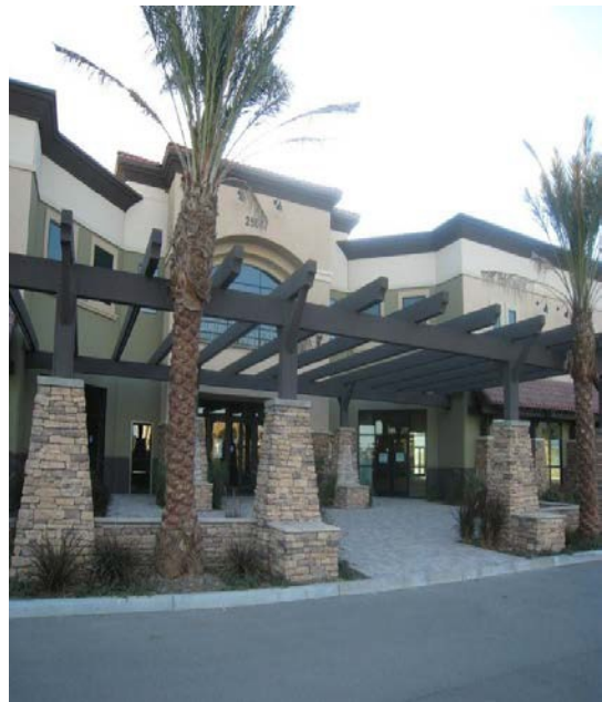
Building Entrances and Access Points
