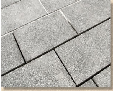
Open Jointed Surface
