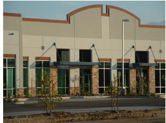
Roofs and Parapet
