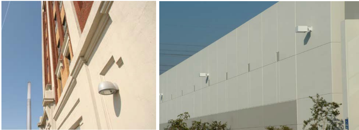
Lighting Fixtures Shield
