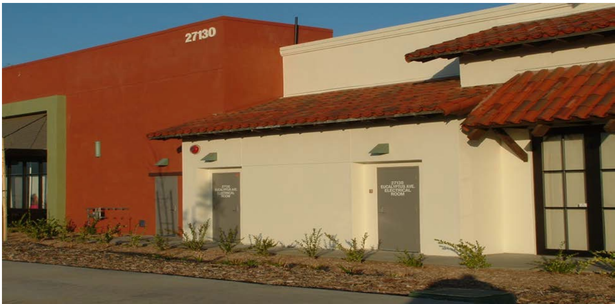
Built in Utility Equipment Room
