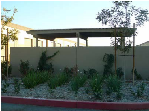
Covered Trash Enclosure
