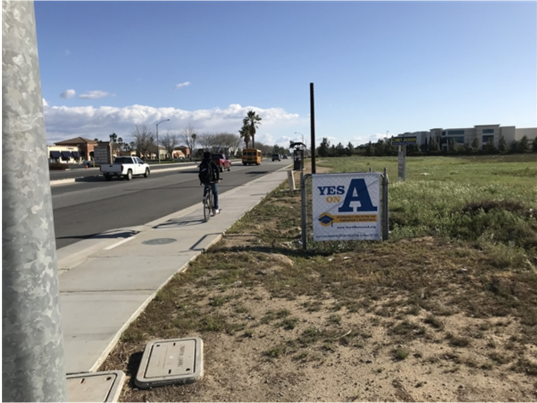
Photo 7: Southern-facing view along the eastern boundary; Perris Blvd is pictured to the left.
