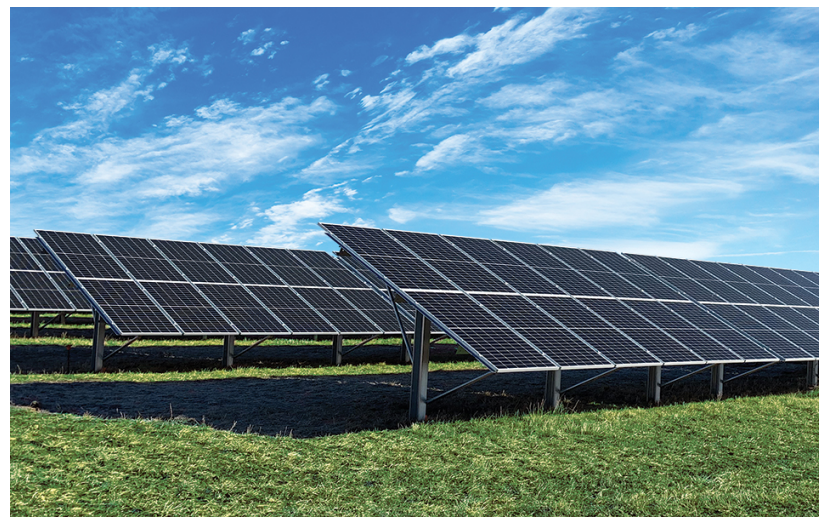
Figure 3-5. Representative Fixed-Tilt PV Trackers
