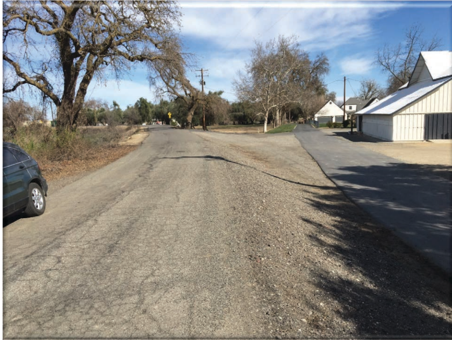
Plate 3. Looking east along County Road 18. The levee rehabilitation project extends from the north shoulder of the road (left side of photo) to approximately 40 feet south of the south shoulder.
