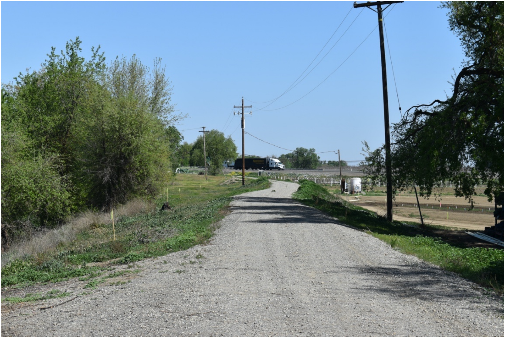
View of eastern-most area of levee restoration project boundary, facing east (April 2021)
