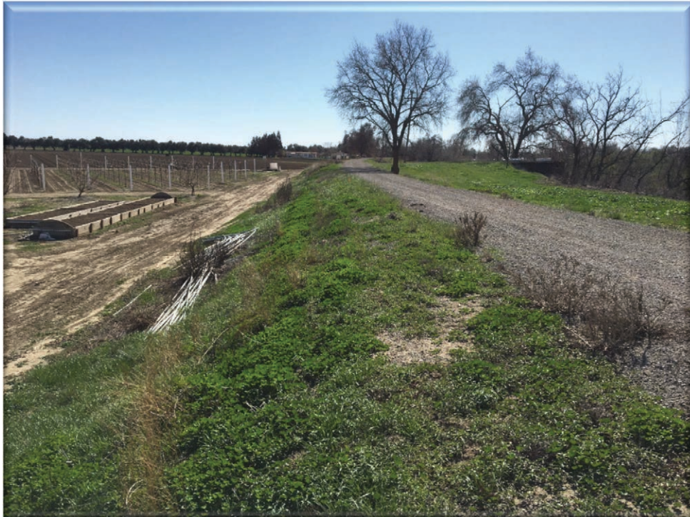
Plate 14. Looking west from Interstate 5 along the levee rehabilitation project corridor. Note the ruderal vegetation along the levee slope between the graveled levee road and the adjacent agricultural field. The valley oak tree along the levee road is also within the project footprint.
