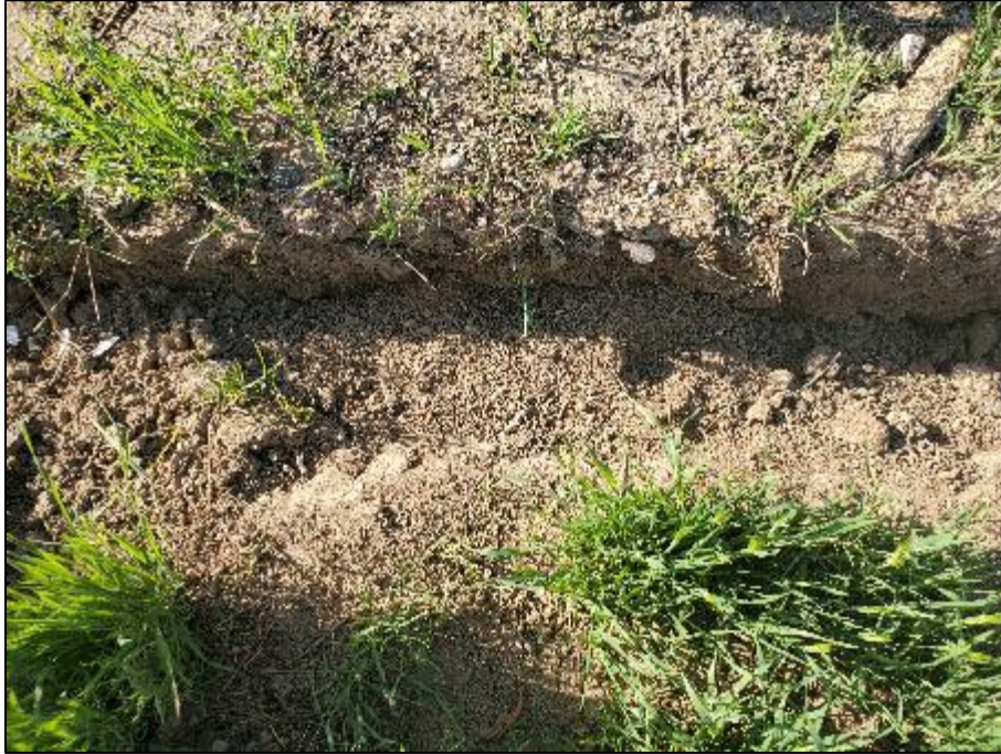
Figure 25. Representative photograph of fence removal, plan view
