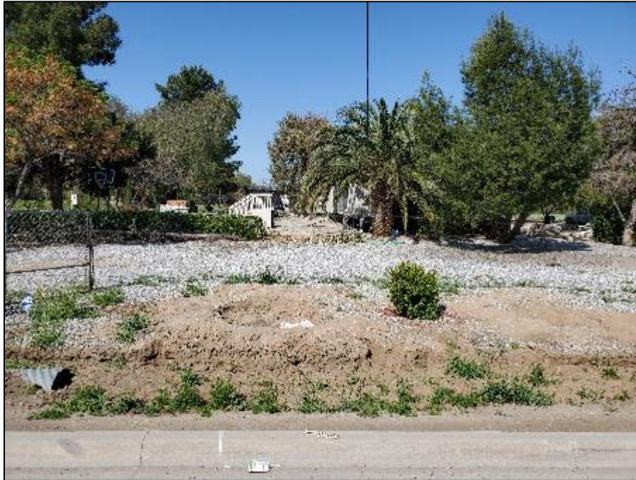
Figure 13. Overview of 3140 Wilson Avenue, view east
