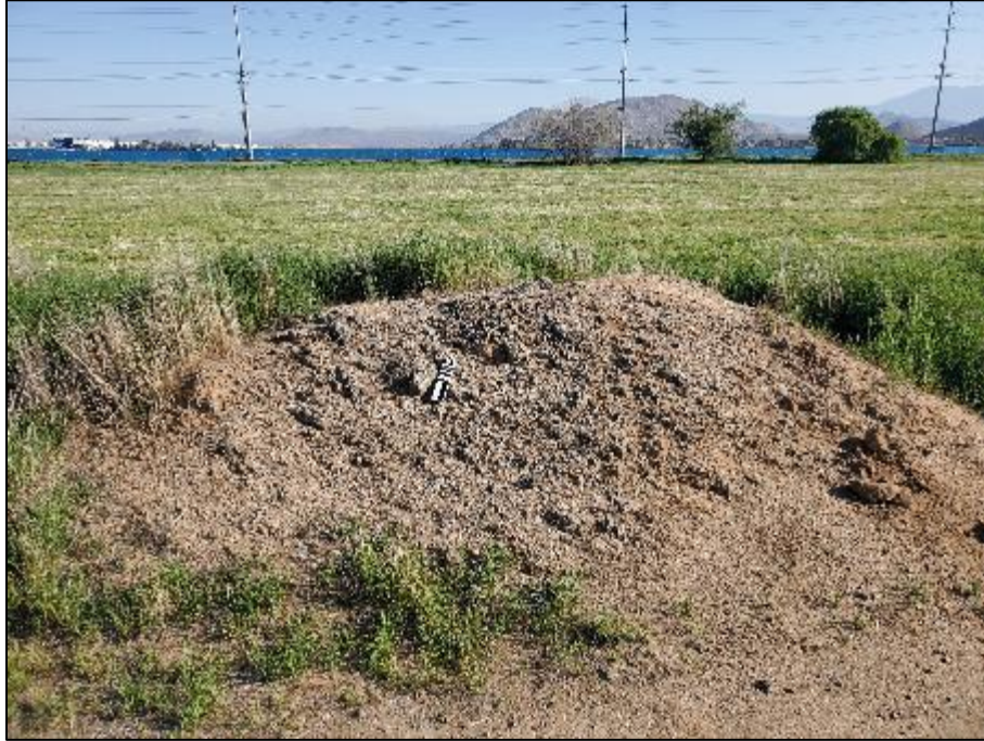
Figure 27. Overview of spoil pile of soil, gravel, and asphalt, view south
