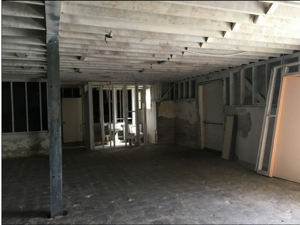
Photo 8: View of former Sunday school room in the basement.
