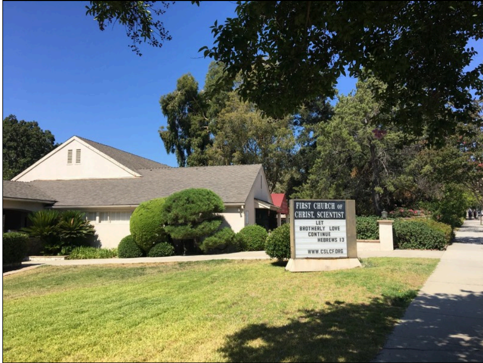
Photo 1: View of north side of the property looking west.
