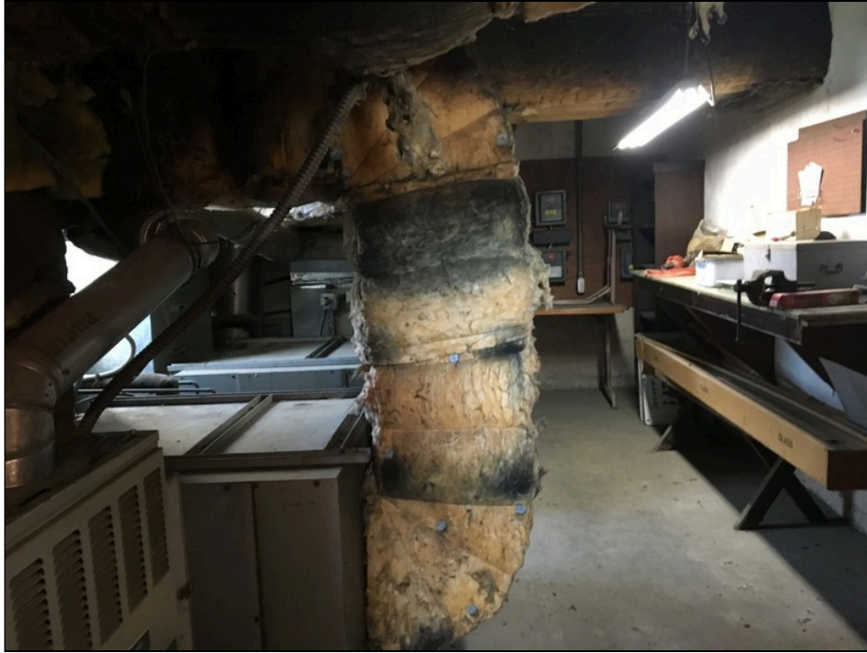
Photo 9: View of furnace room.
