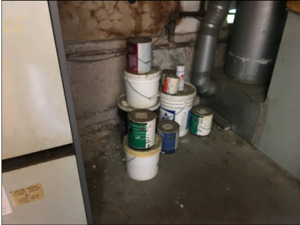
Photo 10: View of paint storage within furnace room.
