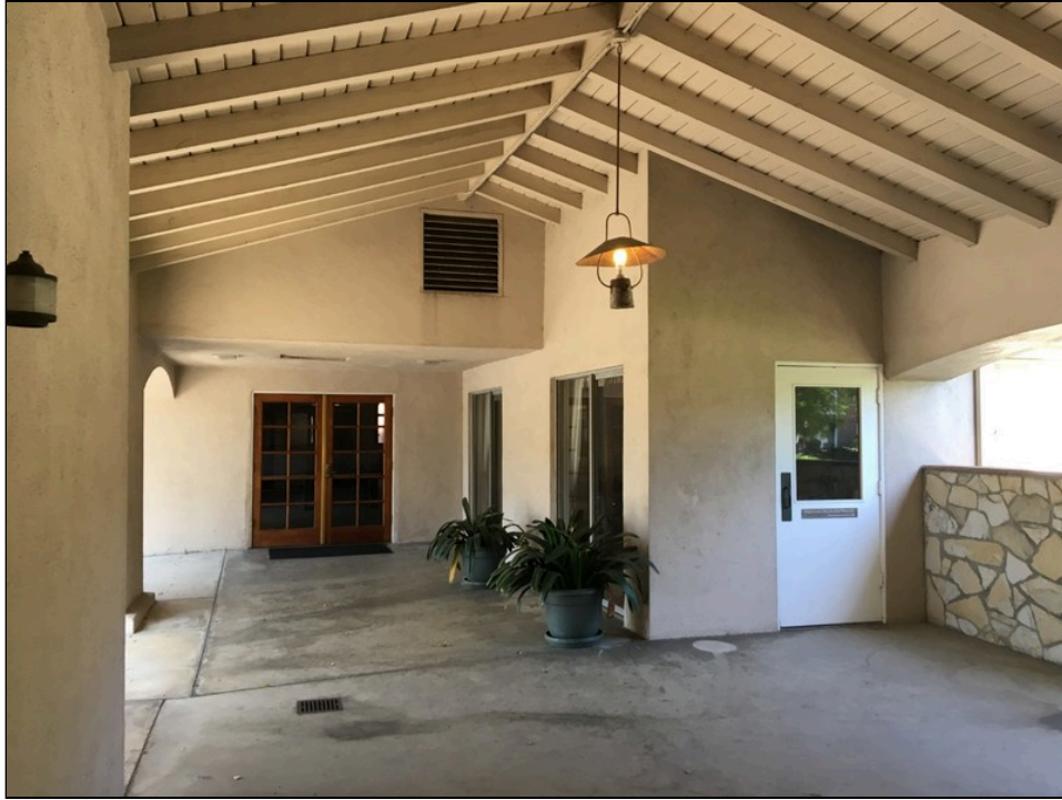
Photo 11: View of exterior walkway between structures and storm drain.
