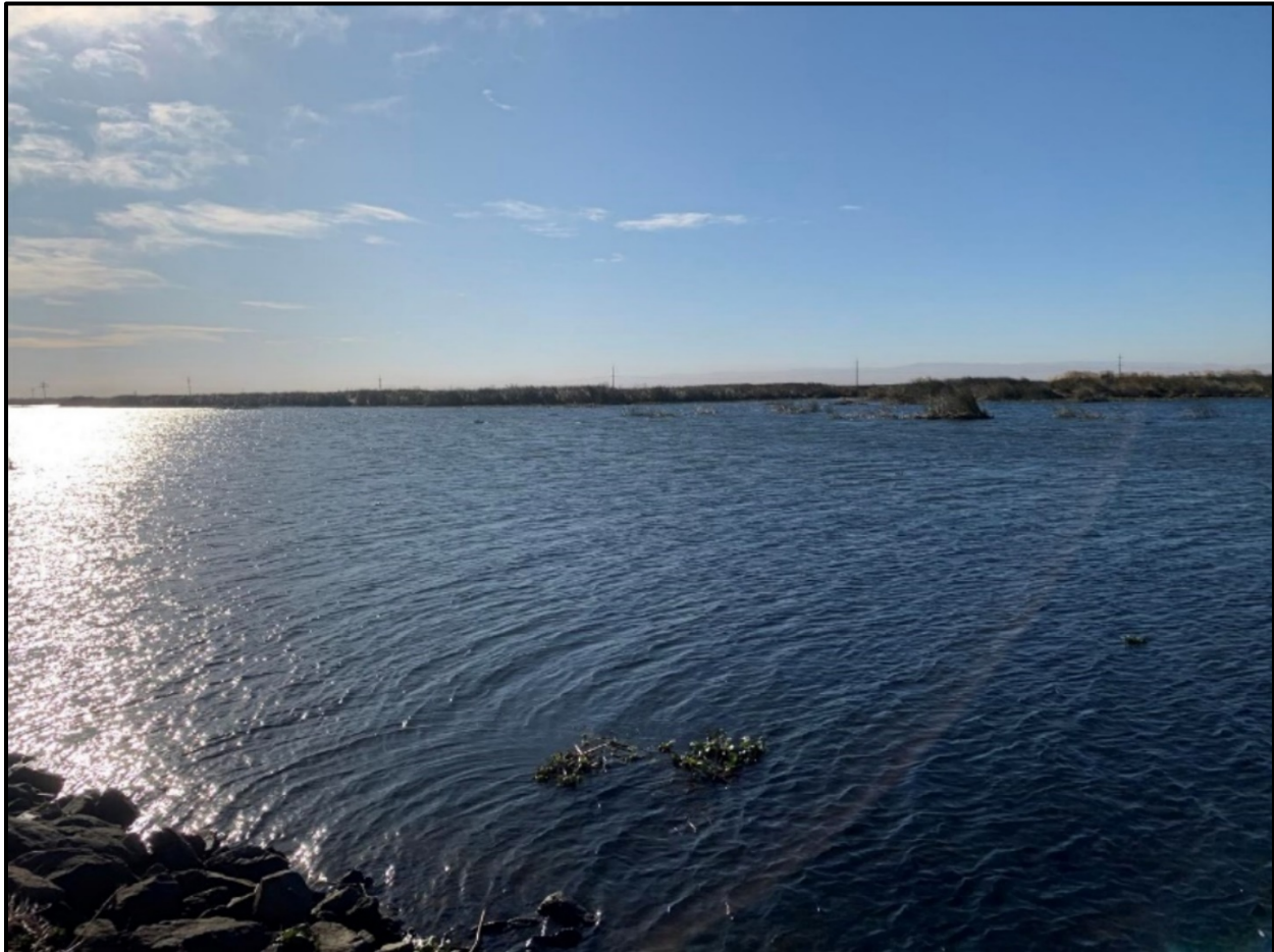
Figure 2-1. View of Segment 1 - Latham Slough from McDonald Island Levee
