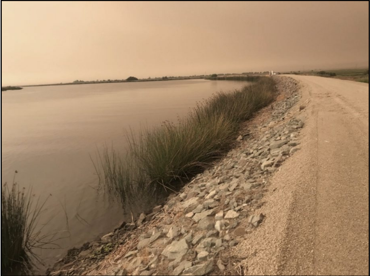
Figure 2-7. Segment 4 – Old River Crossing Location
