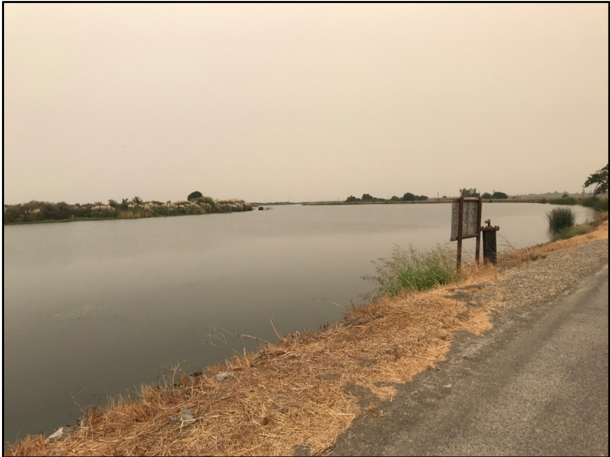
Figure 2-5. Segment 3 – Southeast View of Pipeline Landing on Bacon Island at Middle River Crossing
