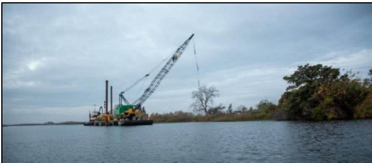
Figure 2-11. Photograph of Derrick Barge from Previous Repair Work at Mildred Island (2019)
