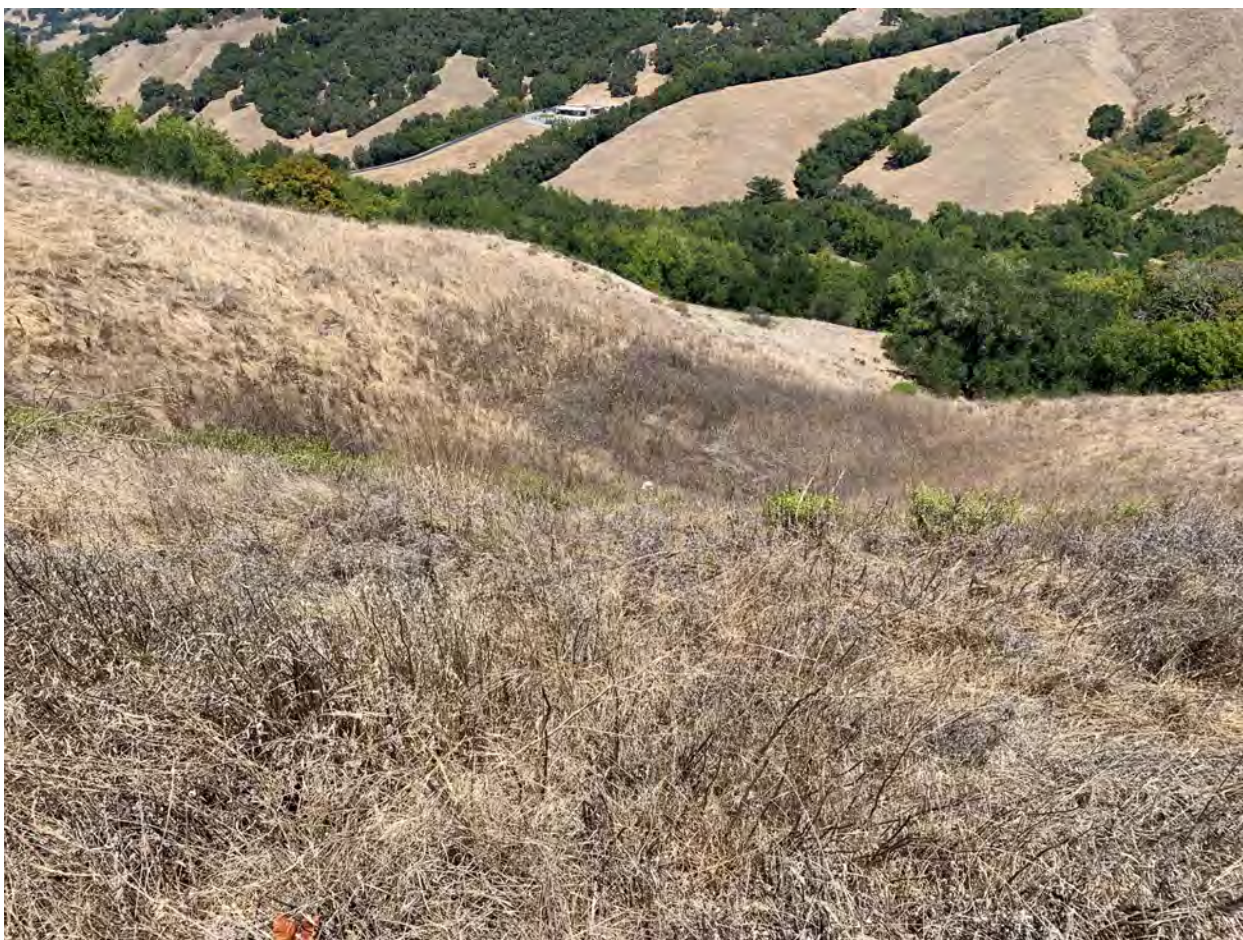
Figure 7: Photograph of landslide below Station 37+00
