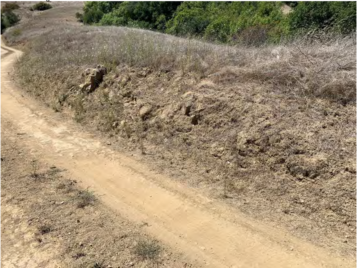
Figure 3: Photograph of existing cut slope at Station 17+00
