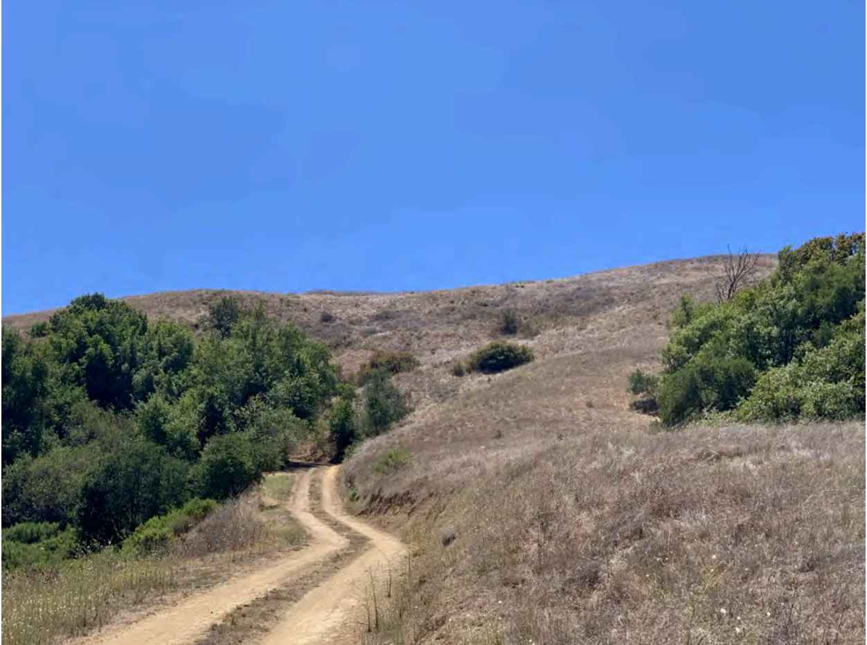
Figure 4: Photograph of mapped landslide above Station 22+00
