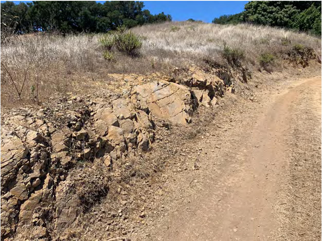
Figure 6: Photograph of cut slopes at Station 37+00
