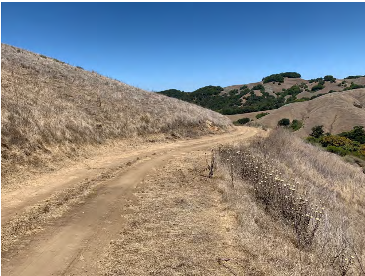
Figure 5: Photograph of roadway at Station 26+00
