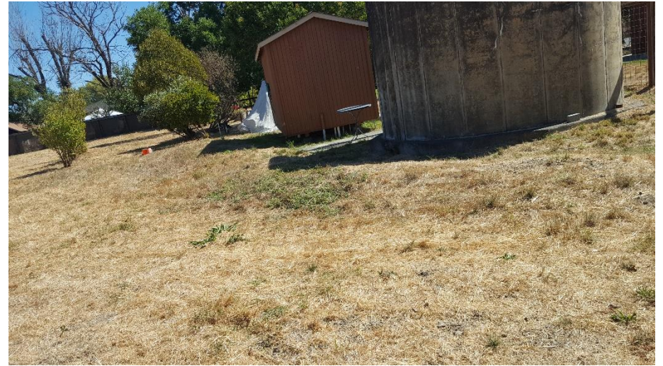
Subject Property - shed & water tank back
