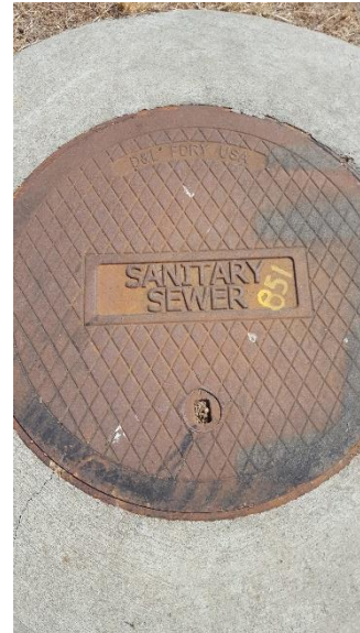
Subject Property - Sewer manhole
